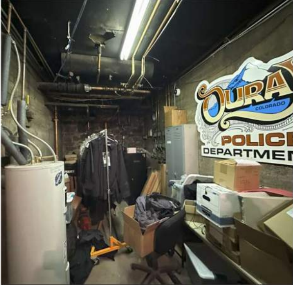
General circulation to the evidence room was obstructed and general storage at capacity, no room to organize
