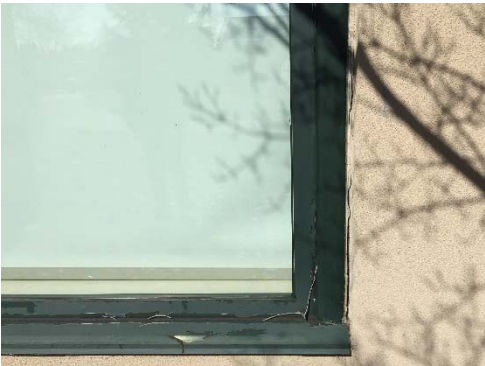
Figure 14: Window at lower level of North House
