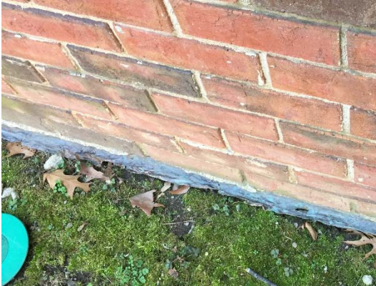
Figure 13: Through wall flashing condition at North House
