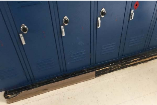
Figure 4: Locker base and baseboard
