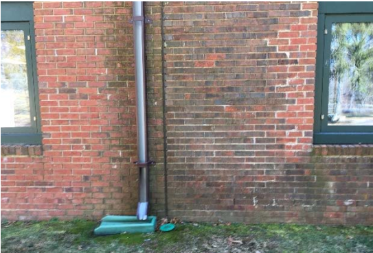
Figure 12: North House masonry conditions
