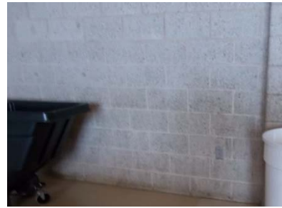
Figure 4: Cafetorium CMU wall
