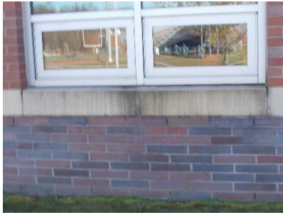
Figure 7: Precast sill
