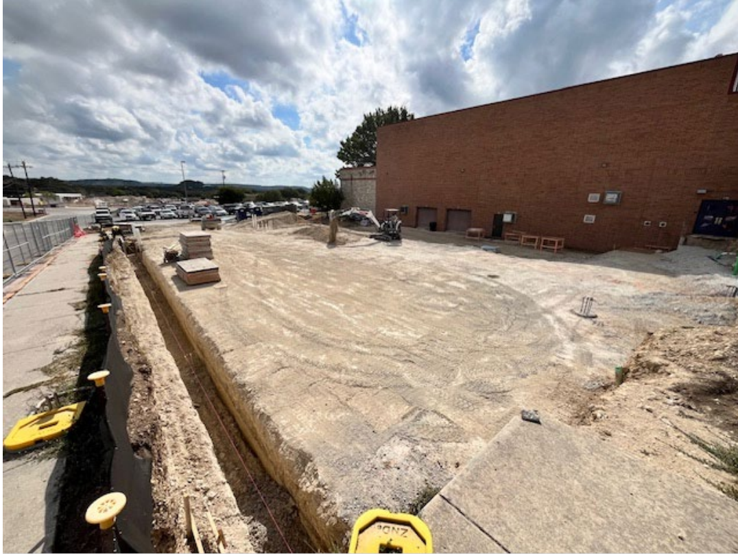
Photo: WHS Weight Room Beam Excavation
