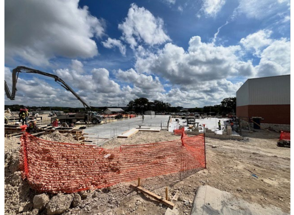
Photo: Slabs/CMU @ Performing Arts
