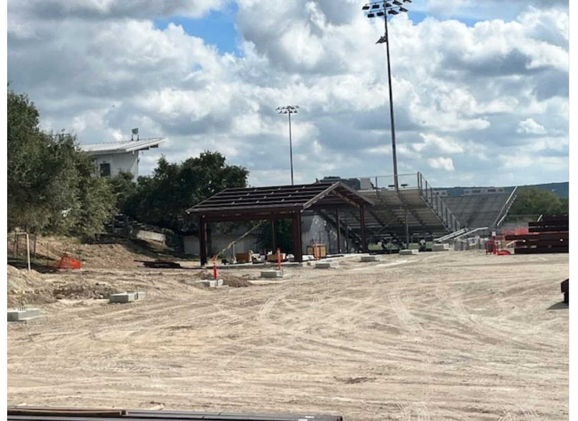
Photo: SMAC Storage Bldg Steel
