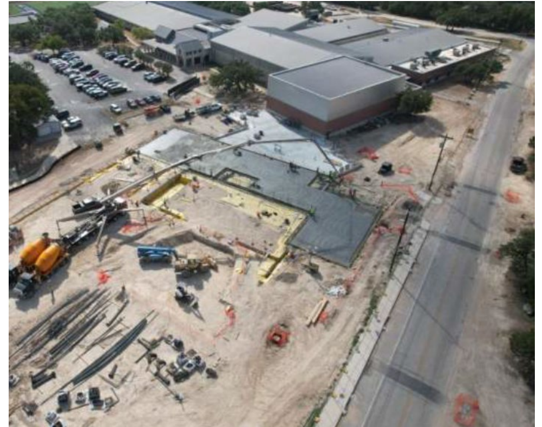
Photo: Concrete Pour @ Performing Arts
