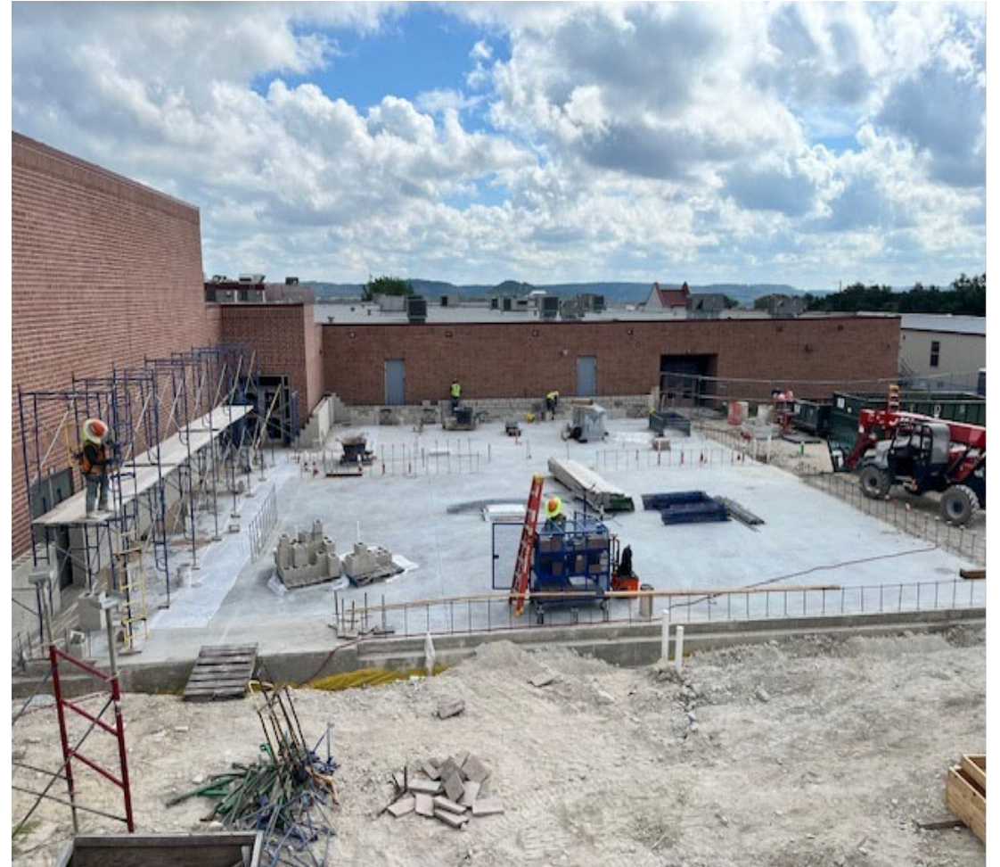
Photo: Band Hall CMU/Slab
