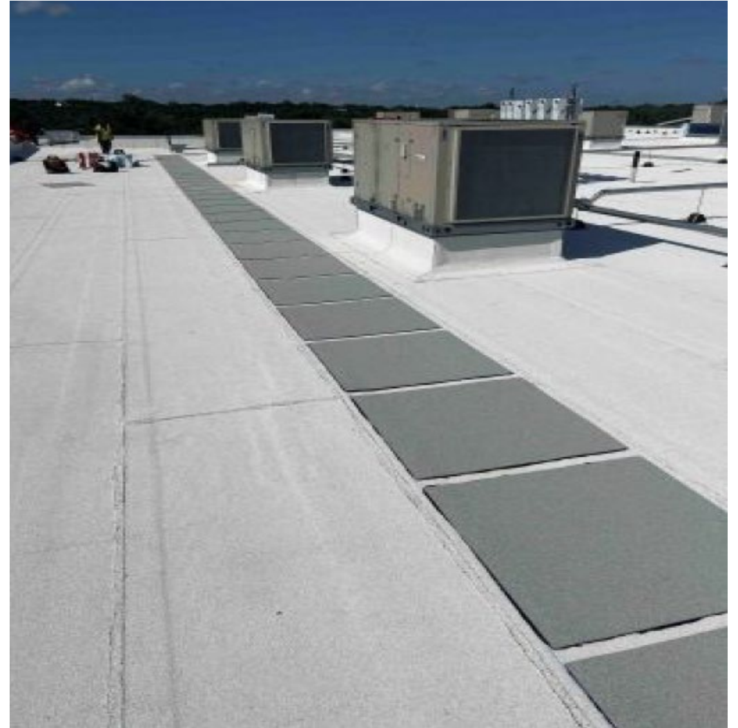
Photo: BHP Roofing
