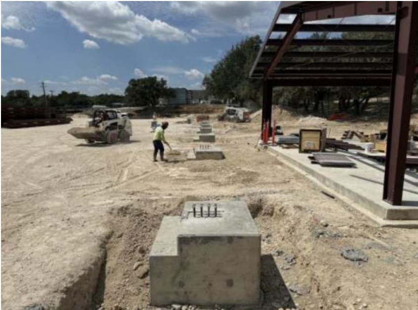
Photo: Pier Caps @ Pavilion
