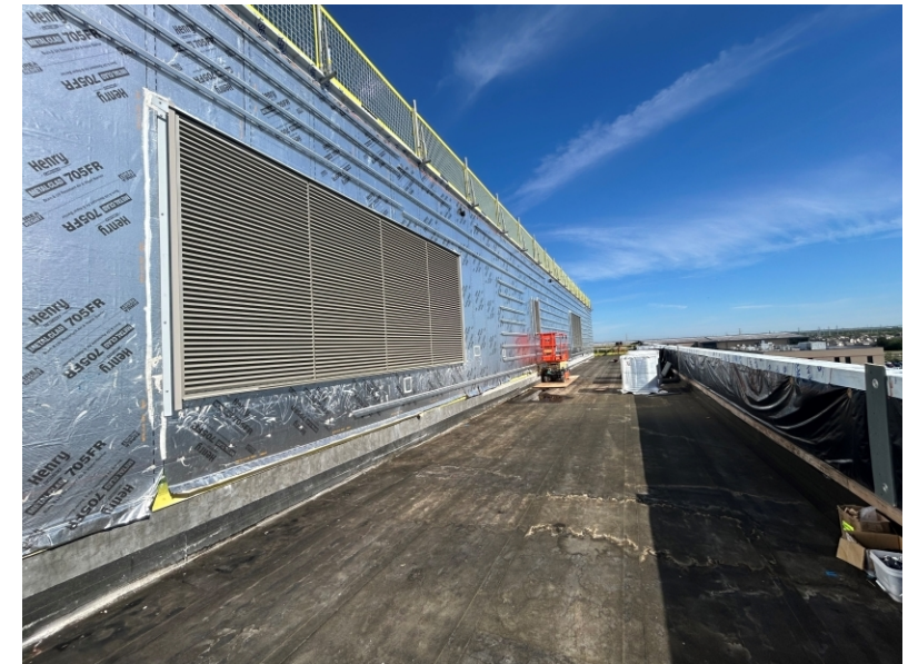
Penthouse louvers placed, metal panel installation in progress.
