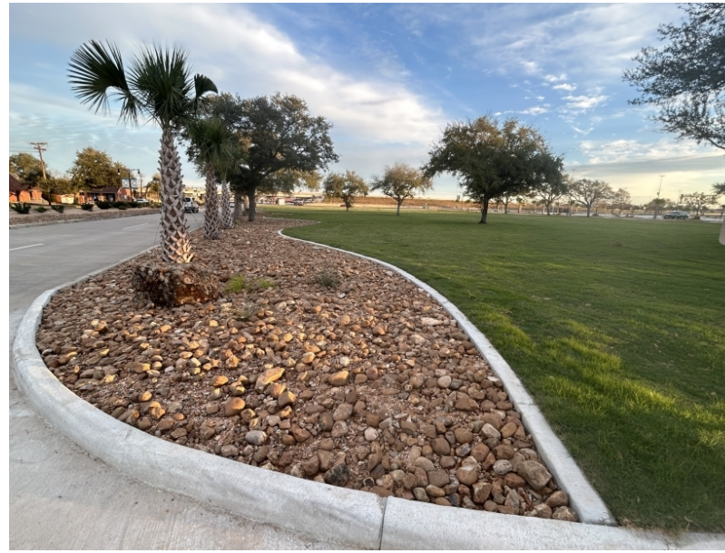
New curb strip at Amburn
