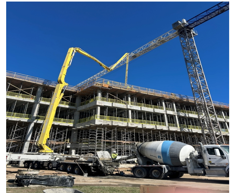
Concrete art roof level area B / C
