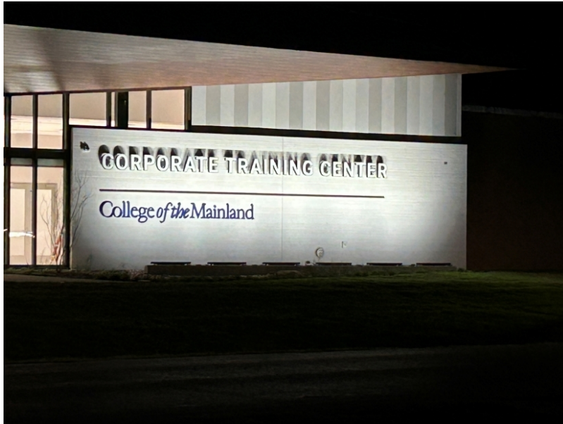
Exterior – Front at night
