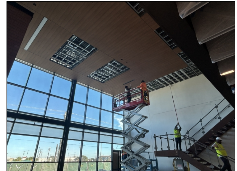
Area A – Ceiling Panels
