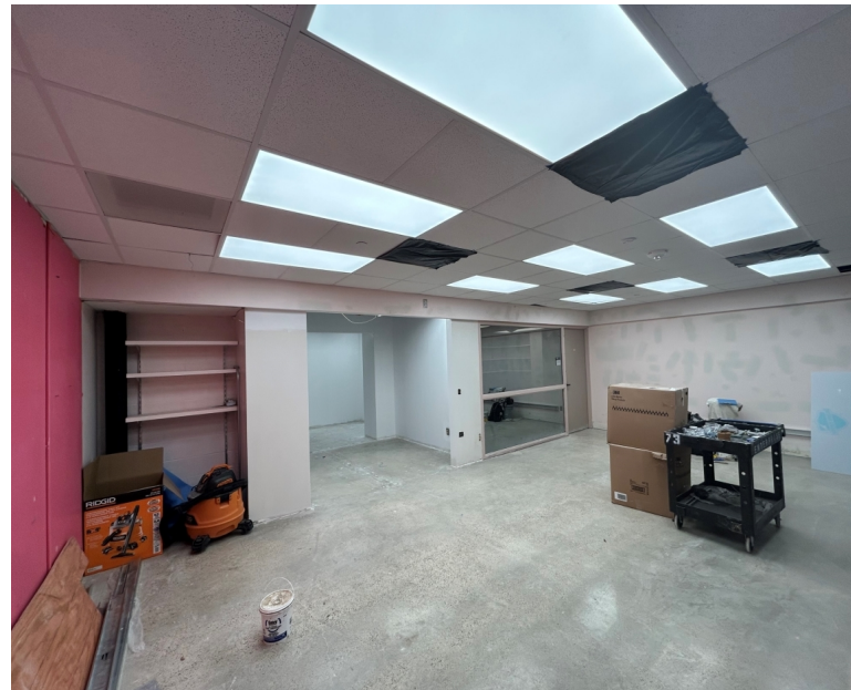
New wall layout and finishes in progress at wardrobe area.
