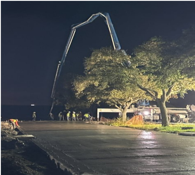
Concrete placement at Lot A in Progress
