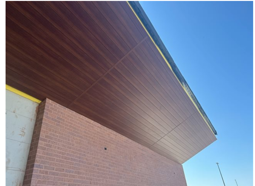
Exterior soffits metal panels in progress
