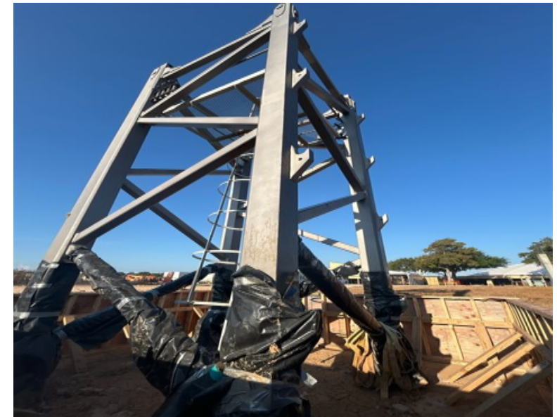
Tower crane foundation, and structure ready to assemble.
