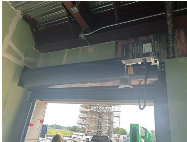
Motorized overhead doors installed at area A
