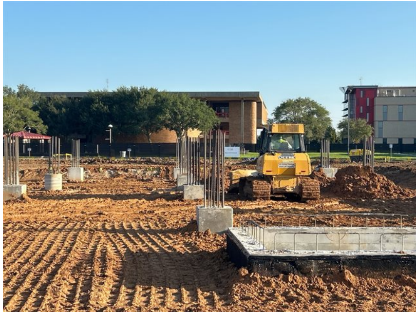
Building footings and column assembly in progress
