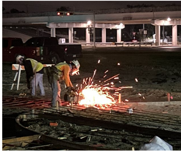
Rebar detailing in progress Lot A
