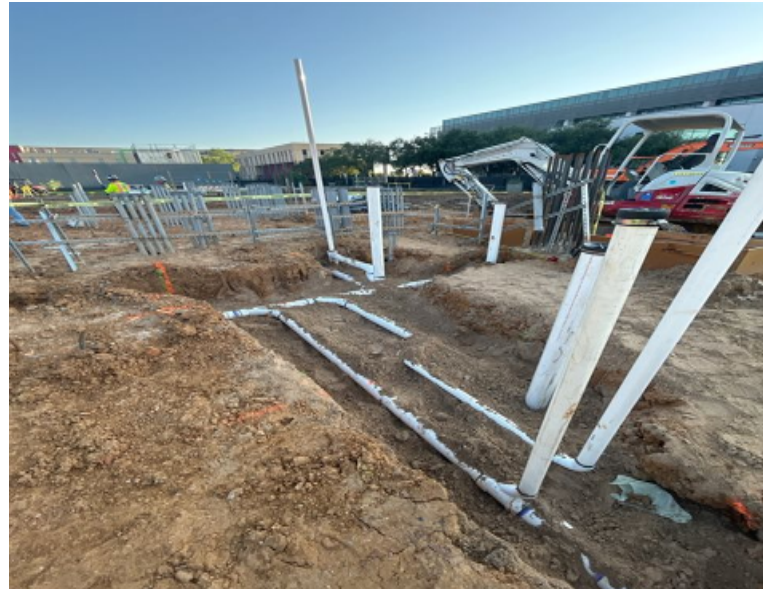
Under slab utilities in progress
