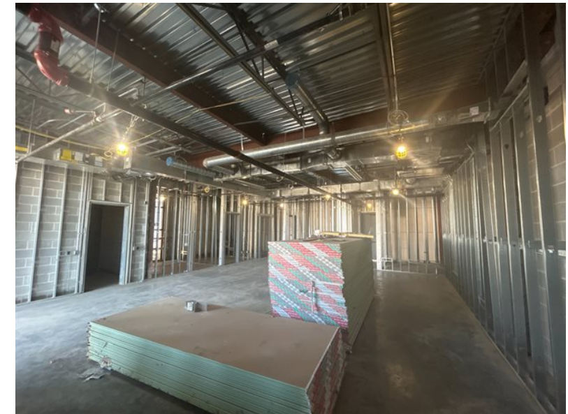
Framing and MEP rough in, complete at area B classroom
