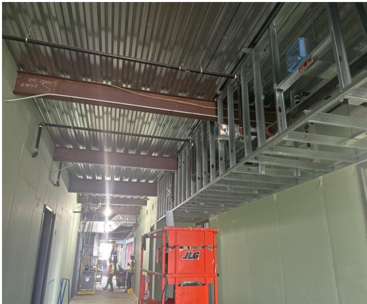
Soffit framing in progress – Area A
