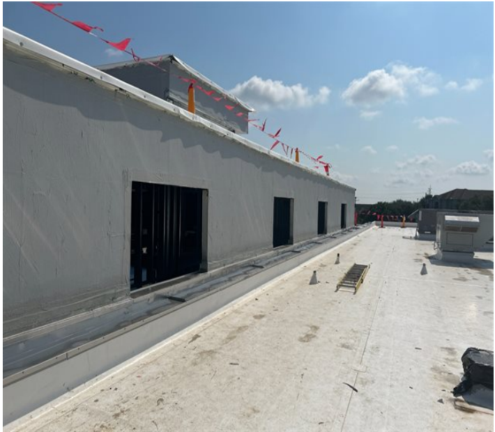
Roof at Welding Addition - Exterior waterproofing in progress.
