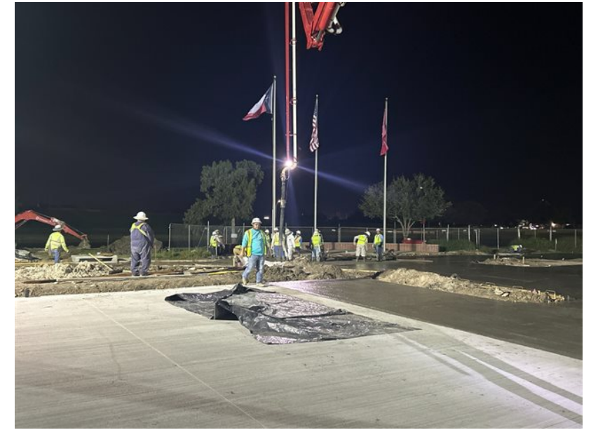
Northern section of Lot A concrete placement
