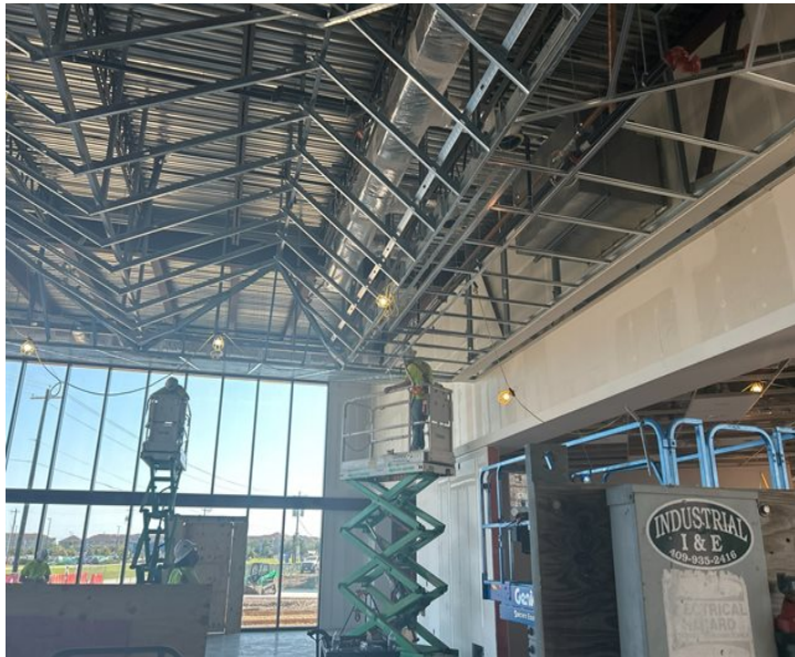
High ceiling framing and MEP's at area A lobby in progress
