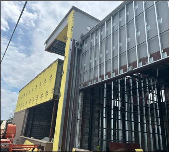
Exterior framing at the Welding Addition
