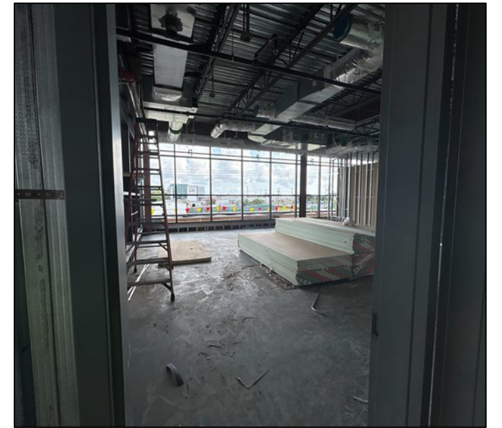
Prep for drywall installation – Area A
