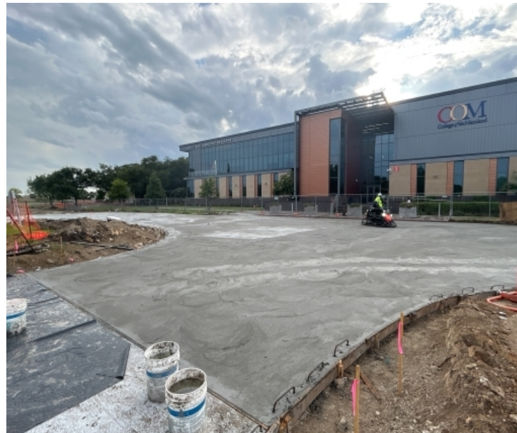
Finishing concrete at Fred Taylor
