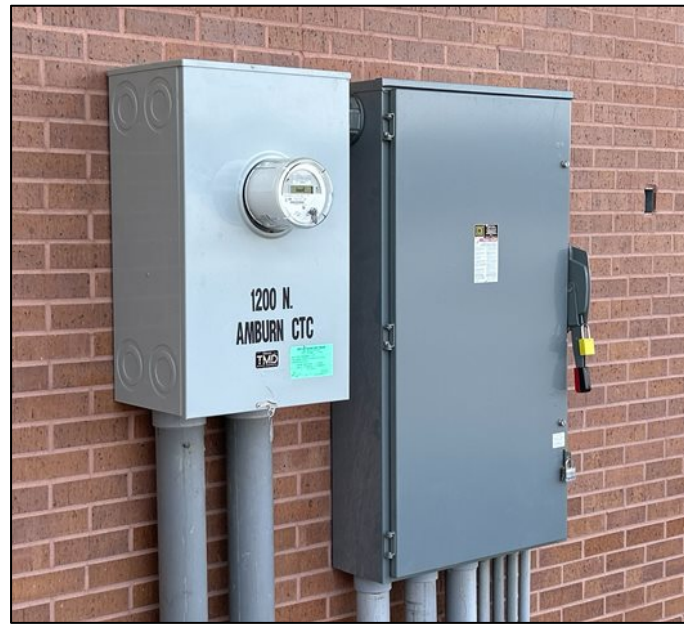
New electric meter installed
