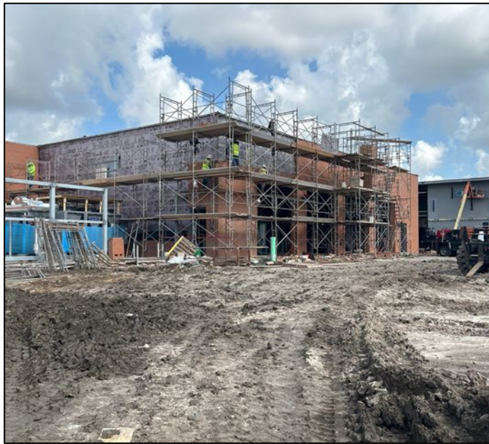
Brick installation – Area A
