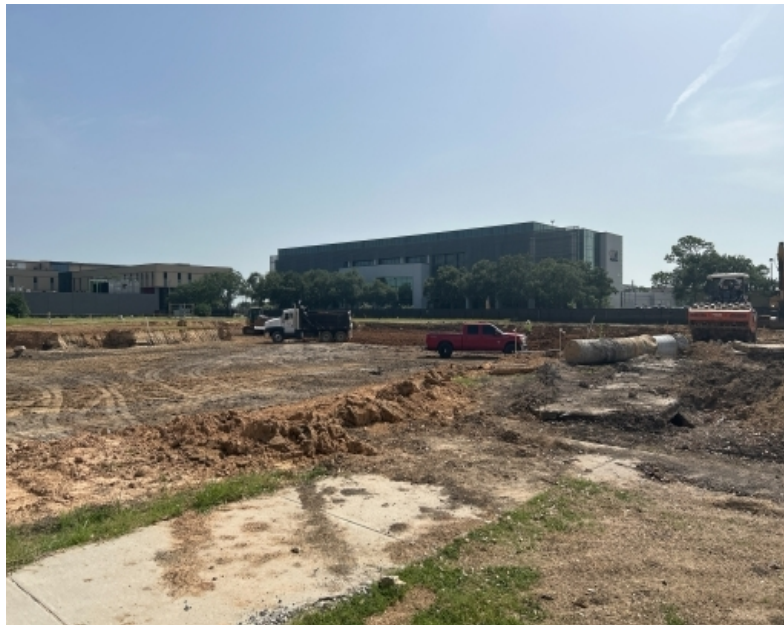
Building footprint excavation complete
