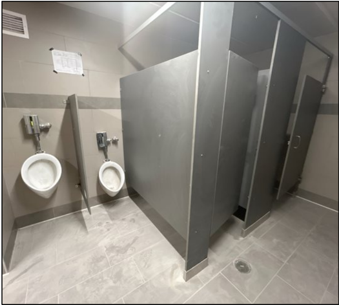
Renovated restroom in the Welding Building
