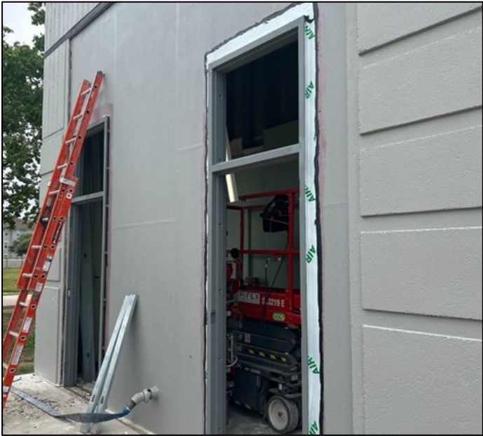
Exterior door frame replacement at the Workforce Education Building
