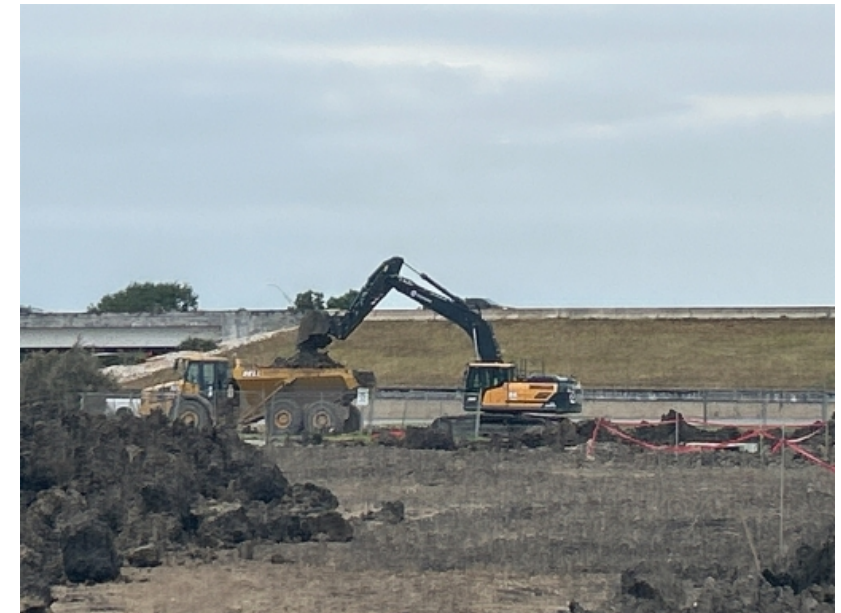
Excavation of Lake Eckert in progress
