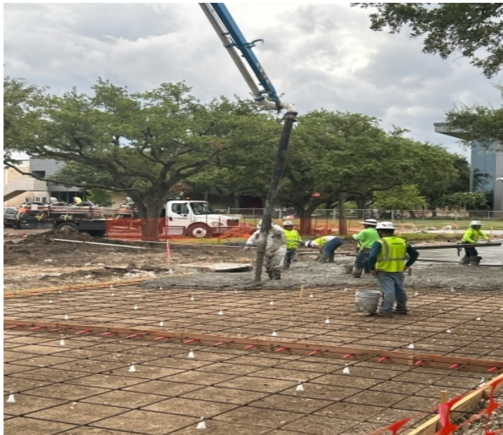
Fred Taylor drive concrete in progress
