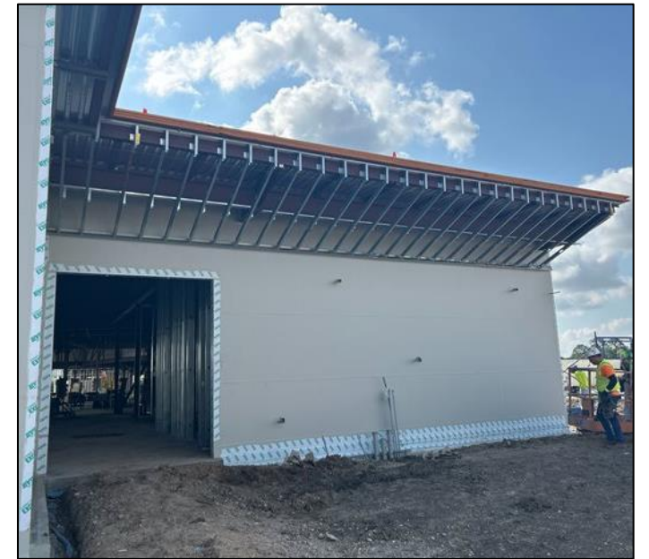
Exterior sheathing and waterproofing
