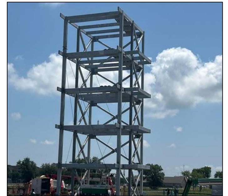
Training Tower structural steel
