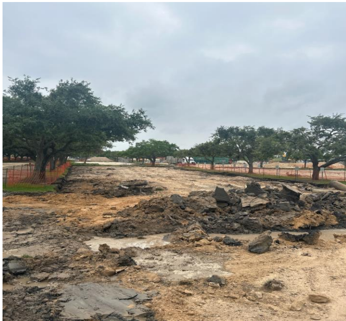
Demolition – Lot A
