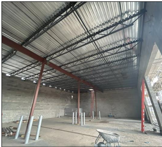
CMU and metal decking at Vehicle Apparatus Bay
