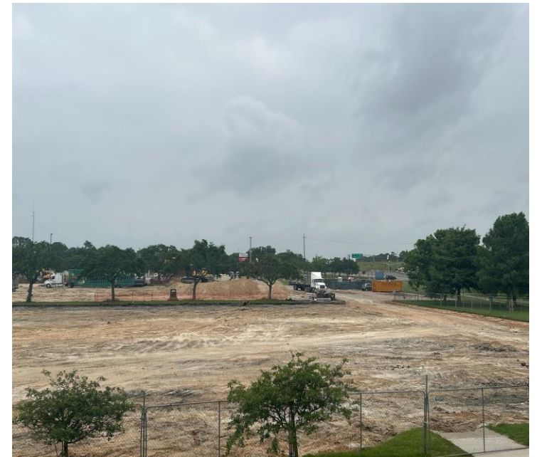
Demolition Lot A
