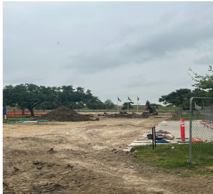
Demolition – Lot A
