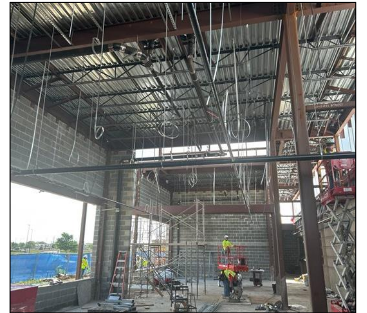
Above ceiling work at Welding Addition
