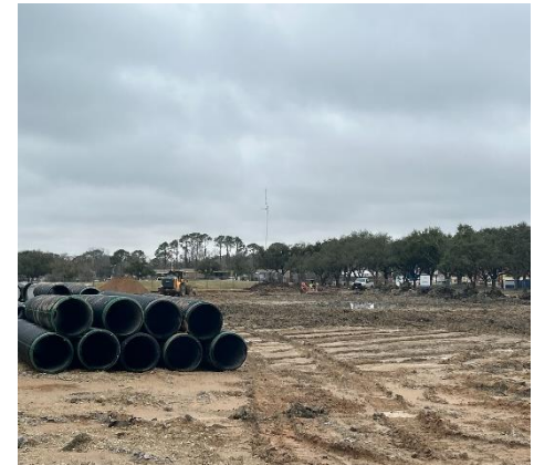
Grading at lot B in progress.
