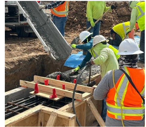
Concrete at grade beams.
