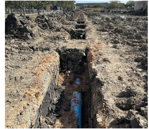
New fire/domestic water in place.
