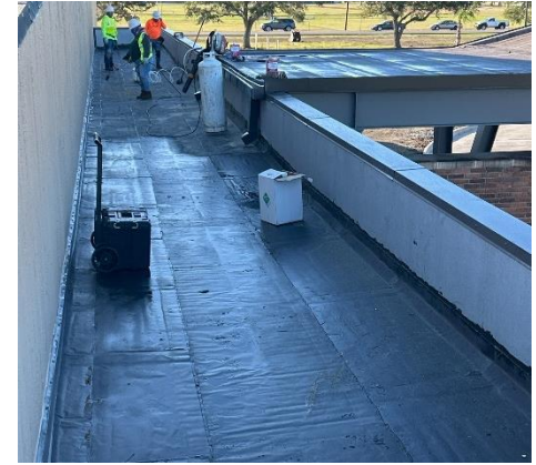
Conf. center low roof in progress.
