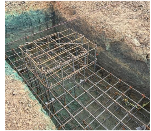
Spread footings reinforcement.
