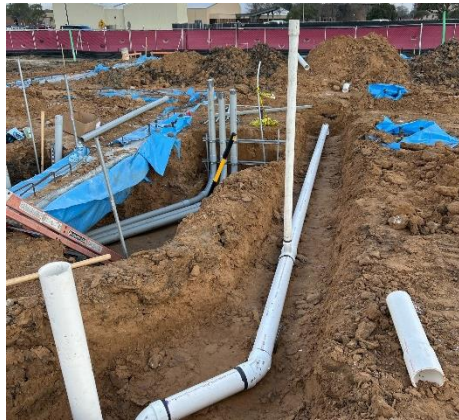
Under slab plumbing in progress.
