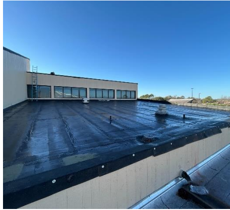
New base sheets installed.
