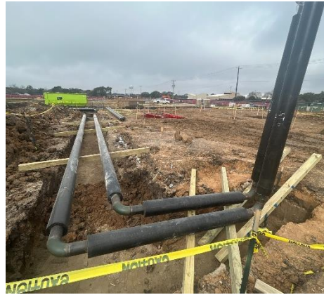
New HVAC system hydronic piping.
