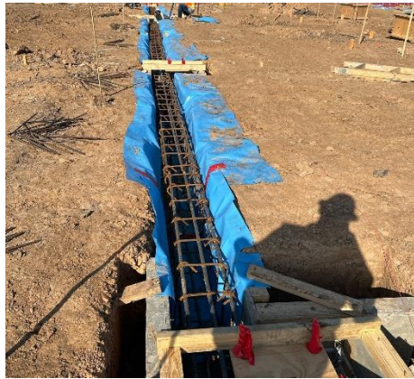
Reinforcement bar at grade beams.
