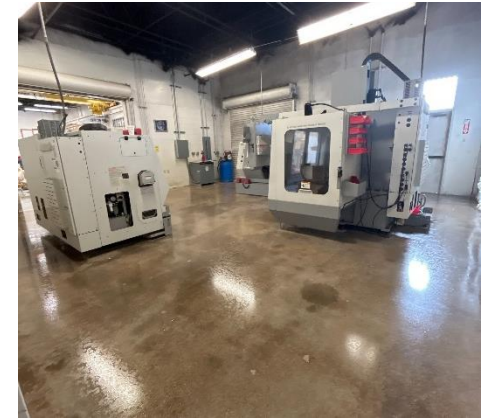
CNC room floor complete.
