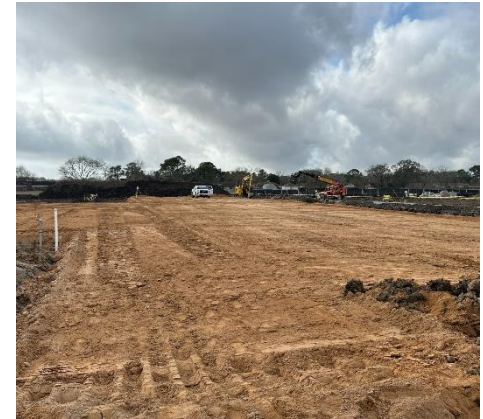
Shooting range building pad complete, survey in progress.
