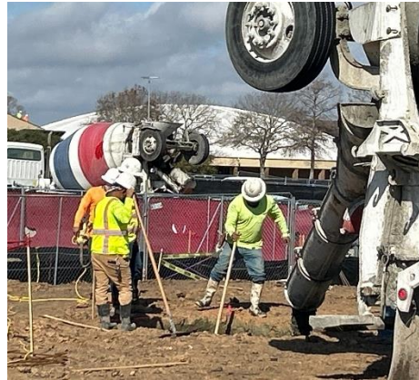
Concrete at spread footings in progress.
