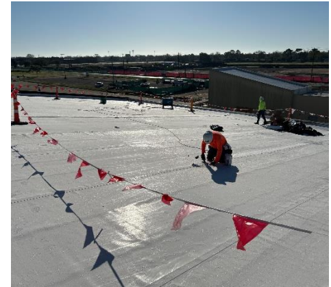
Detail work on top sheet in progress.
