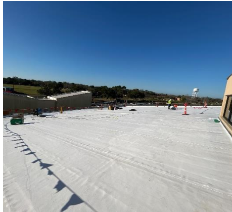
New top sheet in place, working the seams.
