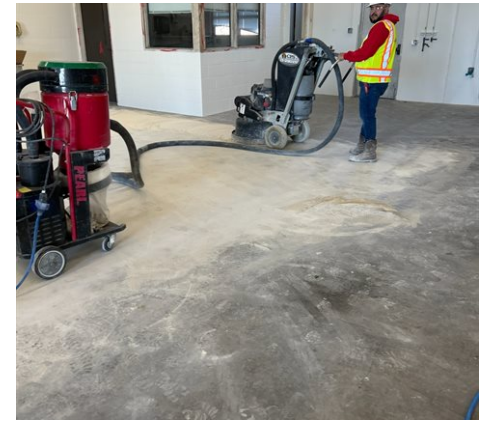
Grinding of existing floor at IE shop.
