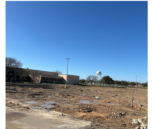
Lot C demolition complete, ready for utilities.
