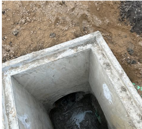
Storm drain inlet boxes in progress.
