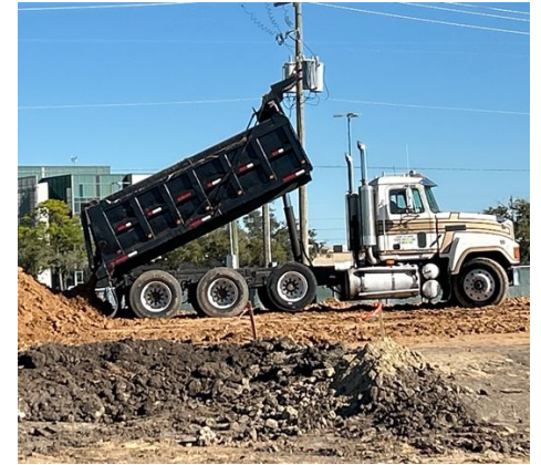
Stabilized dirt delivery for grading.
