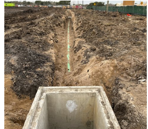
Site storm drainpipe and boxes in progress.
