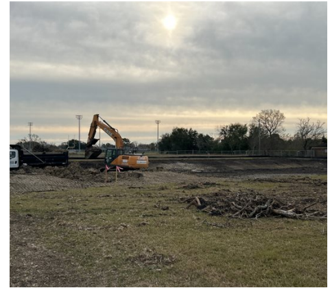
Grading retention pond in progress.
