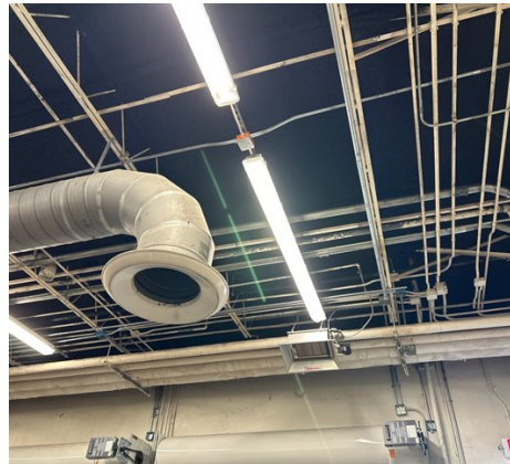
New overhead insulation and utilities at the welding shop, IE building.
