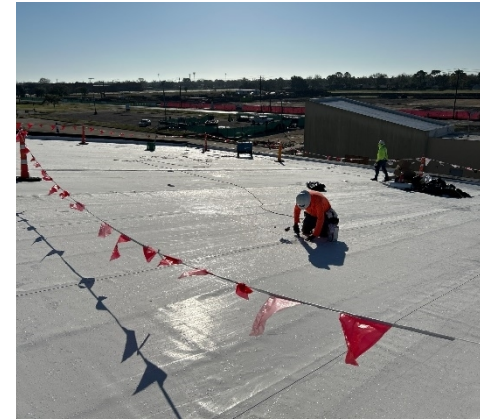
Detail work on top sheet in progress.
