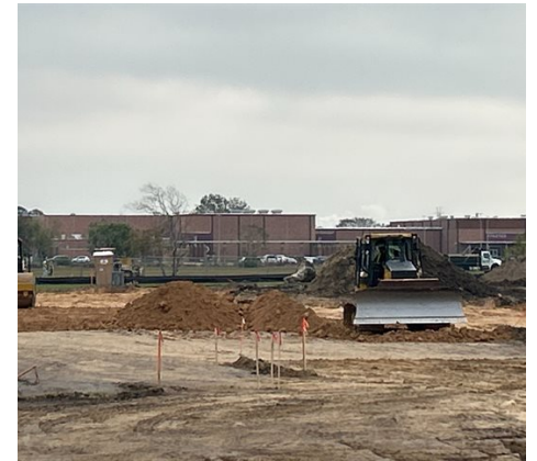
Grading site continues..
