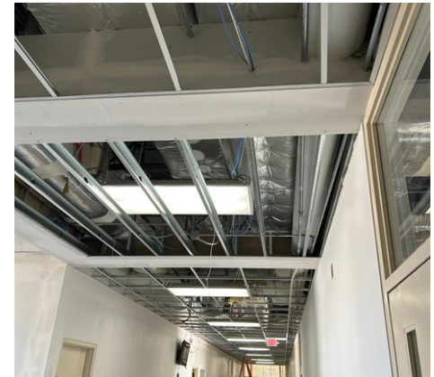
New grid ceiling at the IE building.
