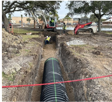
Retention pond final connection..
