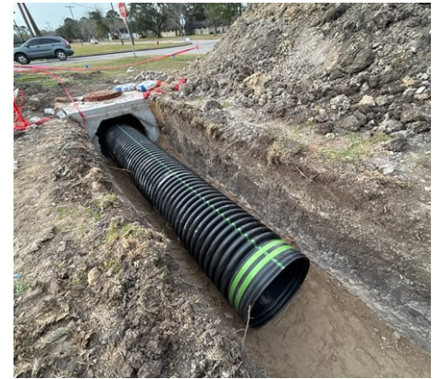
Final storm manhole at lot C.
