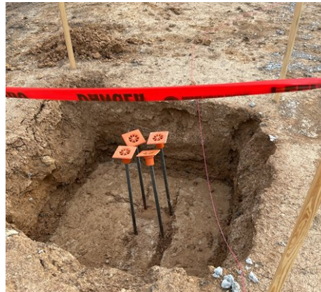
Ready to start grade beam attachment at spread footings.
