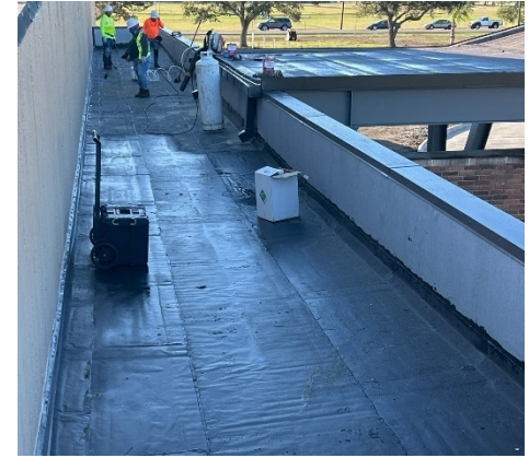
Conf. center low roof in progress.
