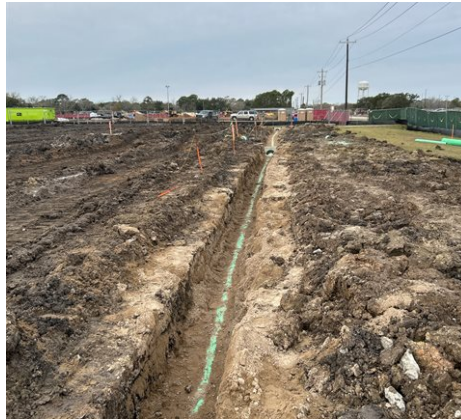
New storm drain pipework.
