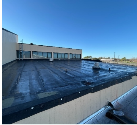
New base sheets installed.
