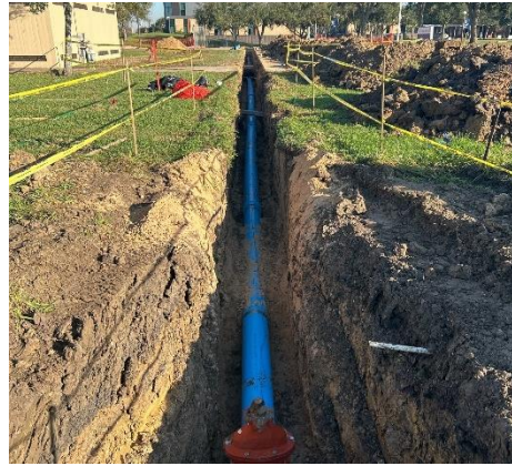
New Fire Water Line Installation
