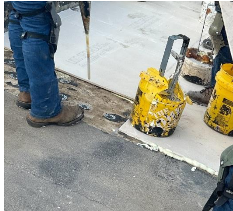
New Fiberboard Installation
