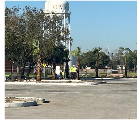
Landscaping In Progress
