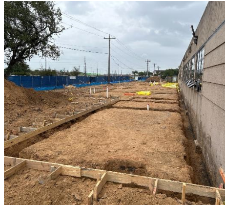
Weld Building Grade Beams Foundation In Progress
