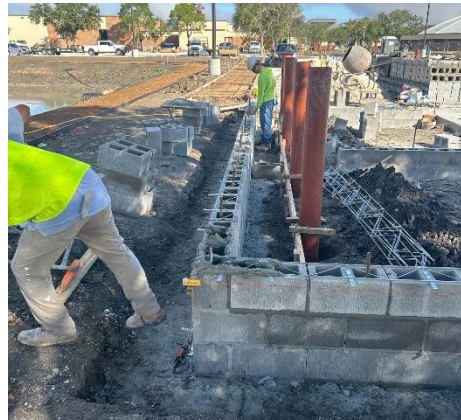
CMU Wall Trash Enclosure In Progress
