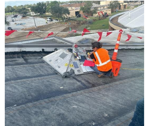
Lift Test In Progress On New Membrane Application
