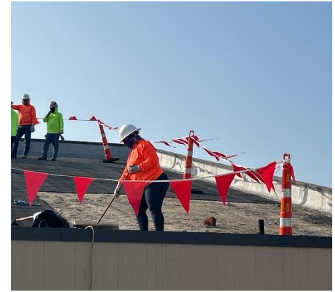
Demolition In Progress
