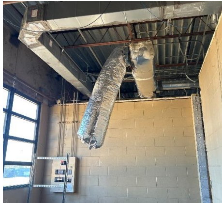
HVAC – New Duct work
