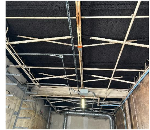
K13 Insulation being applied
