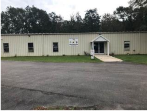
West Elevation Main Entrance
