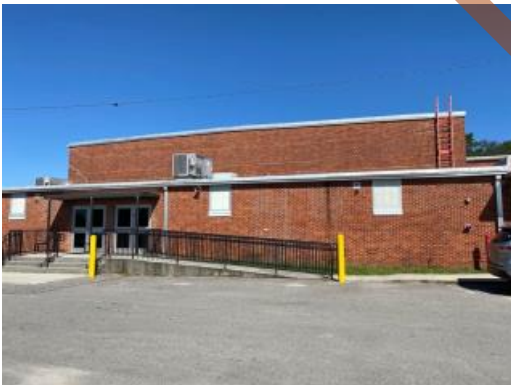
Overall building photo
