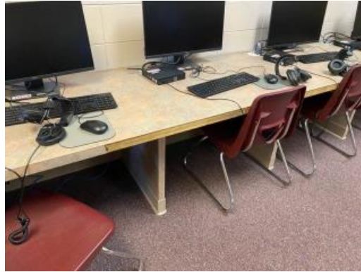
Peeling veneer in computer lab
