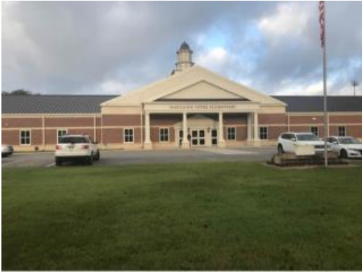
Main entrance Bldg H
