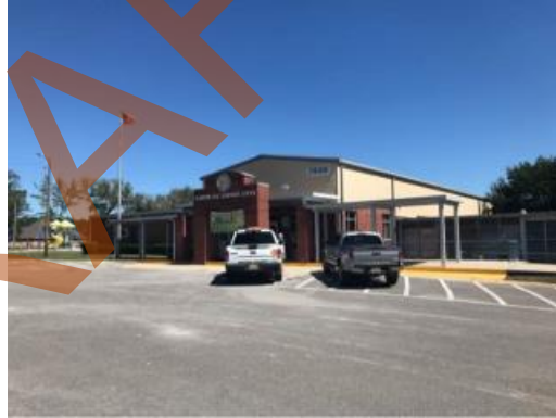
West elevation entrance
