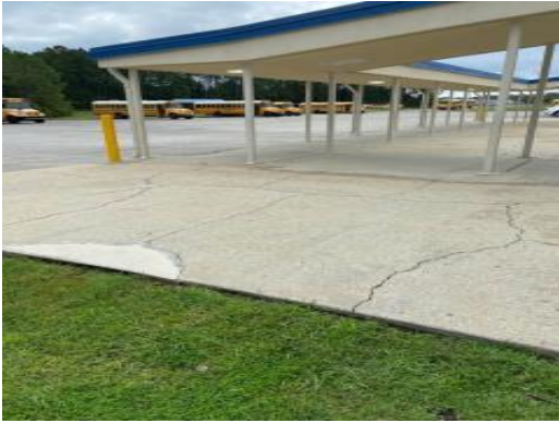
Cracked sidewalks
