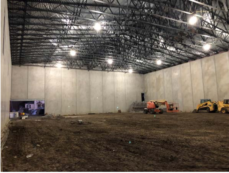
Gymnasium interior looking east
