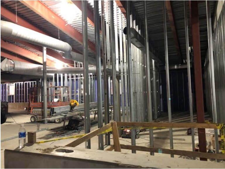
Commons light gauge framing at men's restroom
