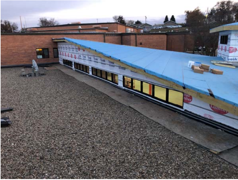
Commons clerestory windows above existing middle school roof
