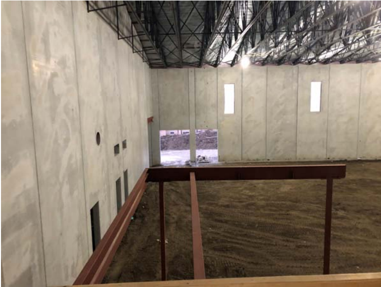
Steel framing at mezzanine adjacent to elevator
