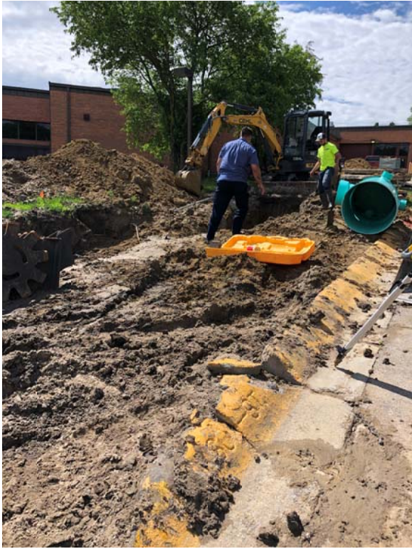
South end of main storm sewer being installed
