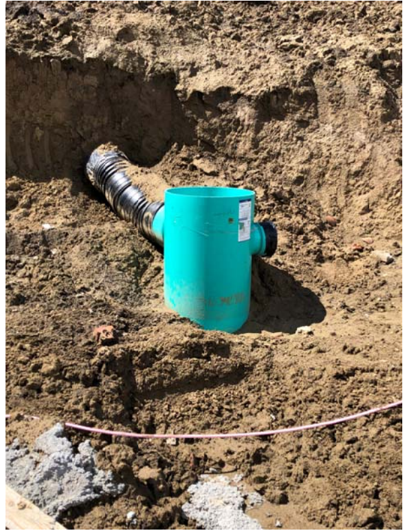
Existing storm sewer rerouted
