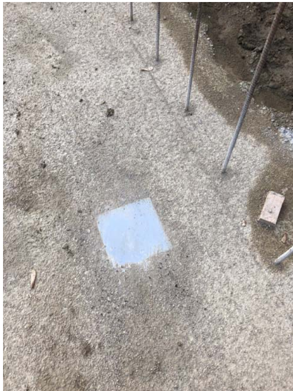
Steel embed for precast panels
