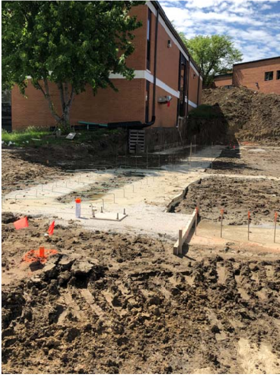
Footings for East wall of Gymnasium
