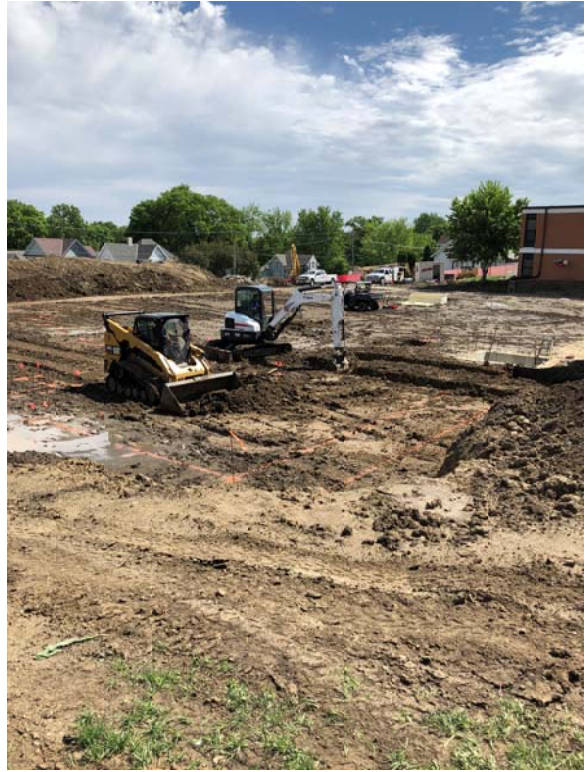
Digging footings west of elevator pit
