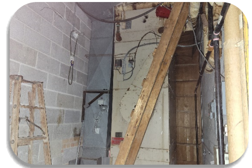
Gold Gym AHU, circa 1967 (Offline, Typical of Two) – Demo in Place
