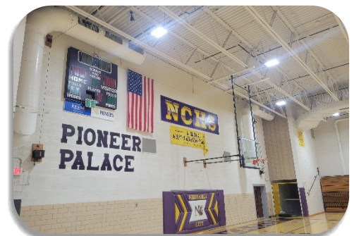
High School Gold Gym Heat Pump Ductwork – Remove and Replace
