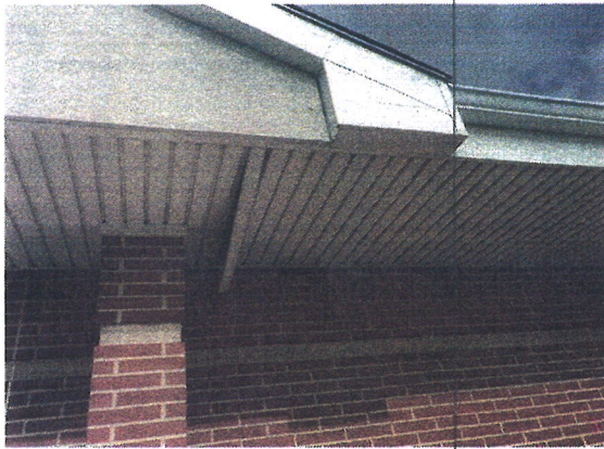
East Elevation Soffit
