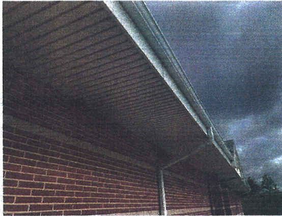
East Elevation Soffit
