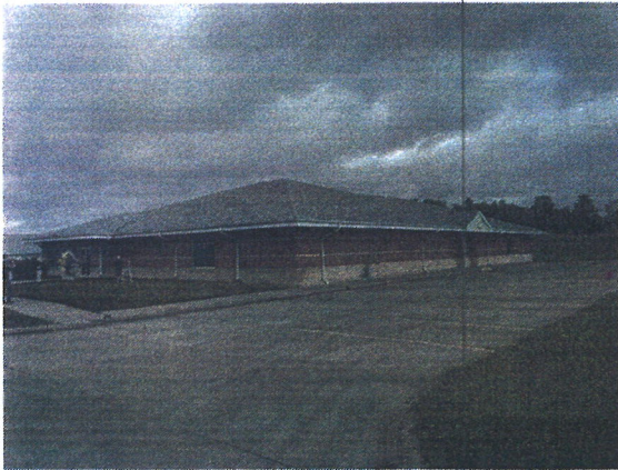
East Elevation Overview
