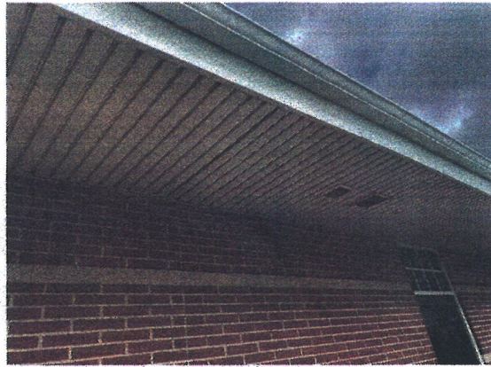
East Elevation Soffits
