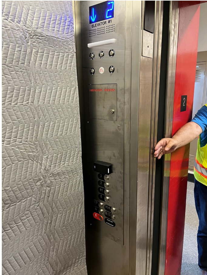
New elevator cab and mechanicals
