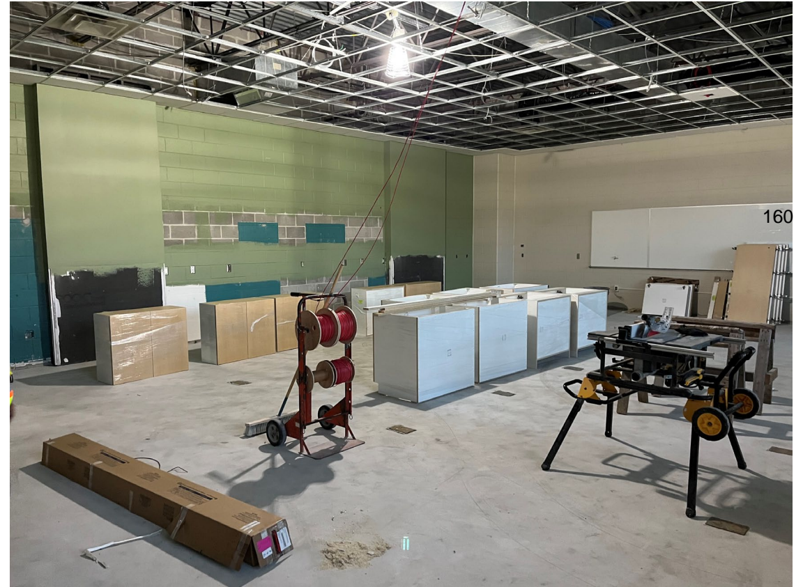
Extensive renovations in Art Room
