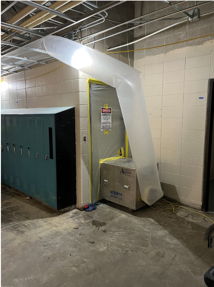
Locker rooms are now being abated
