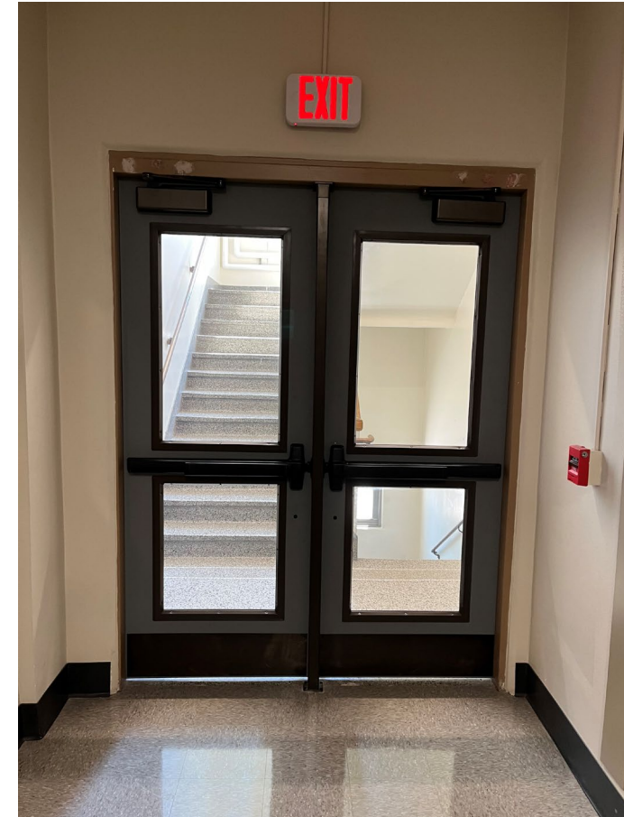
New fire doors at all stairwells
