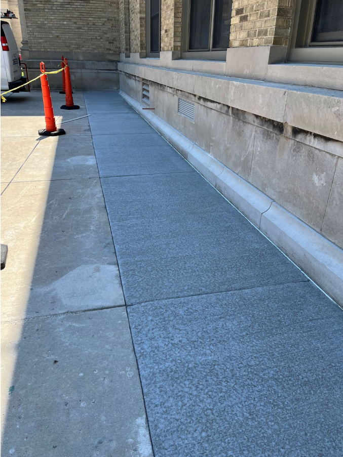
Replaced limestone and concrete plaza at Arts & Sciences
