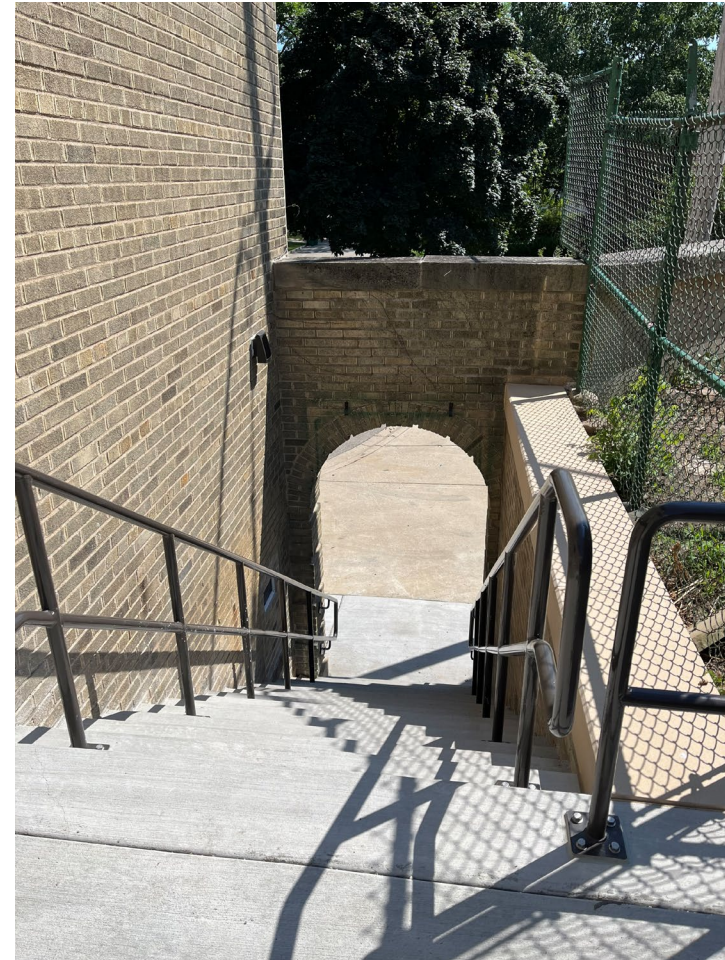
Walkway open to the public again
