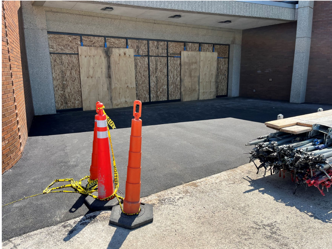
Below grade waterproofing and hardscape at track entry
