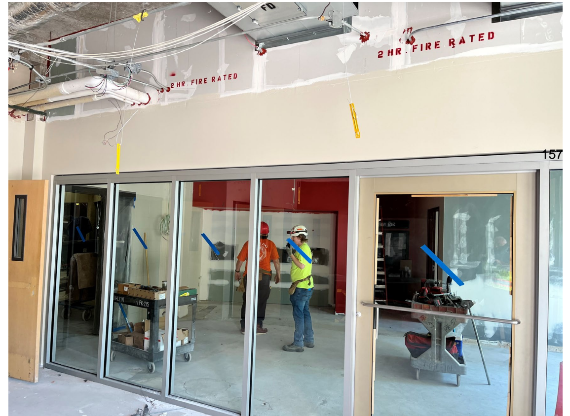
Main entry and administrative office suite
