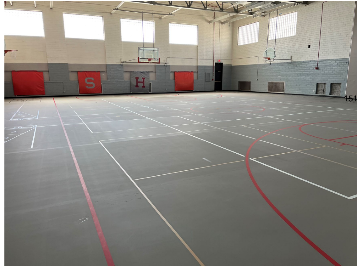
New flooring is complete at North Gym
