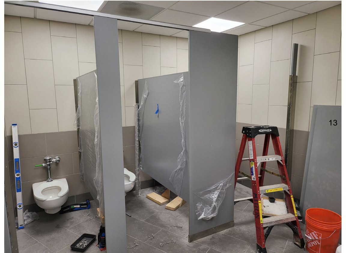
Renovated restrooms nearing completion
