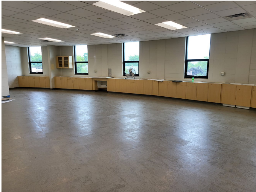
New casework installed in classroom
