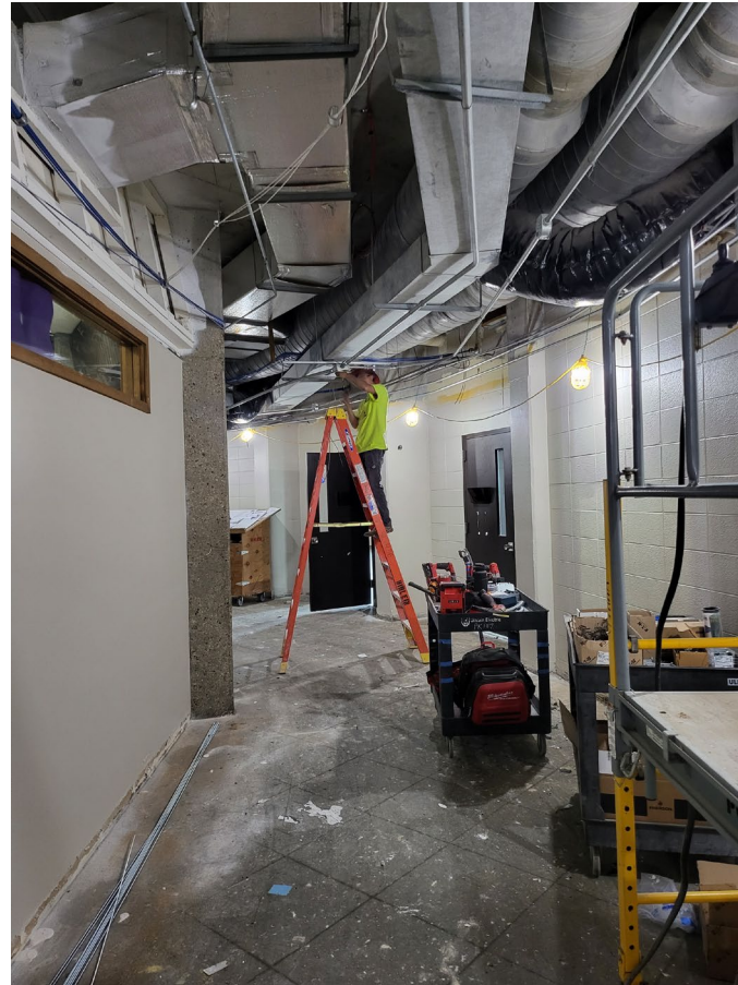
Ductwork improvement throughout corridors
