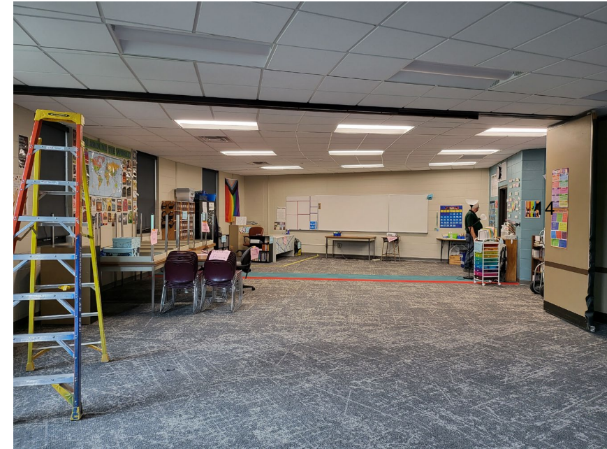
Renovated classroom with wall dividers
