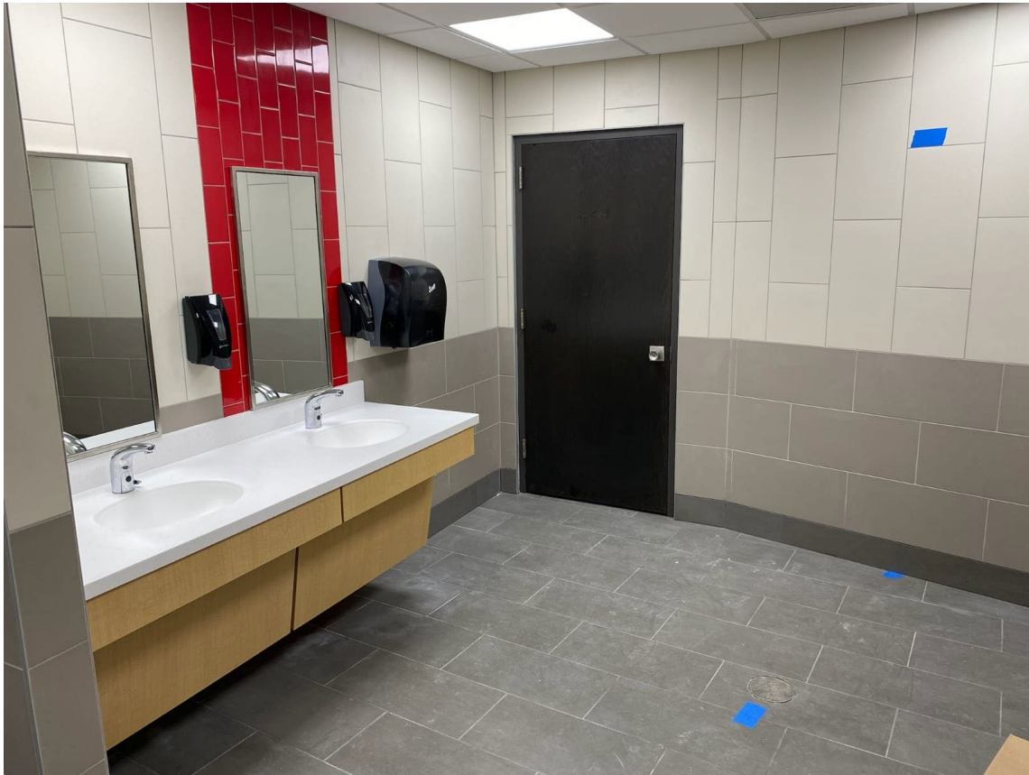
Boy's Bathroom almost complete
