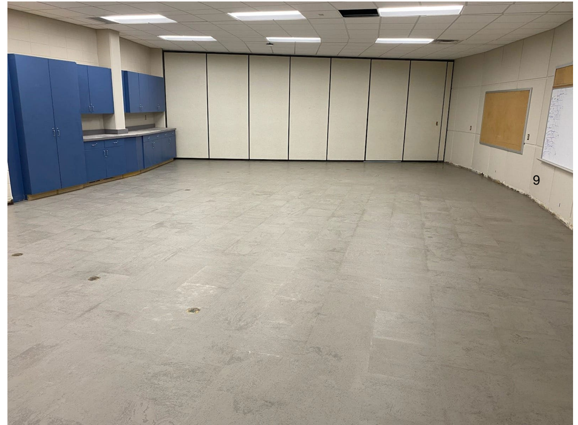
Classroom 110 almost finished
