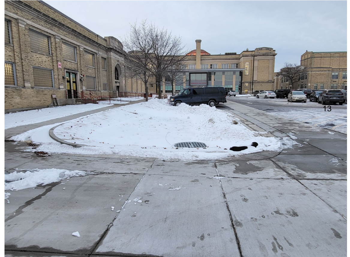
Bioretention basins are complete
