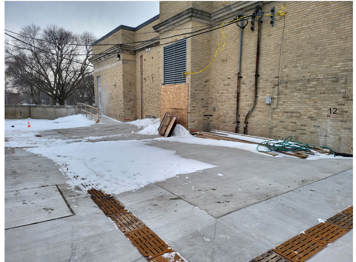
New ADA access ramp (in background)
