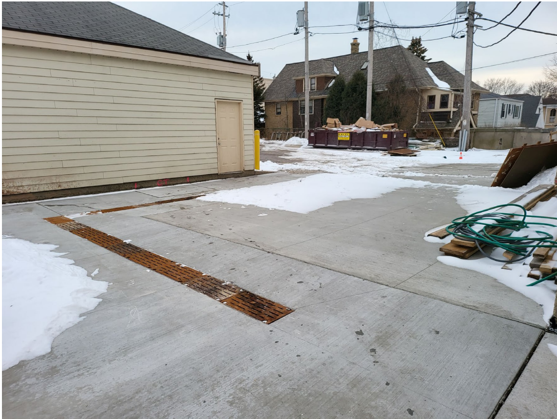
Concrete cap over lower-level structure
