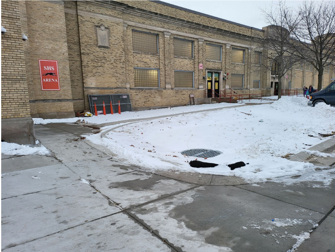
Improved stormwater management at Arena entry
