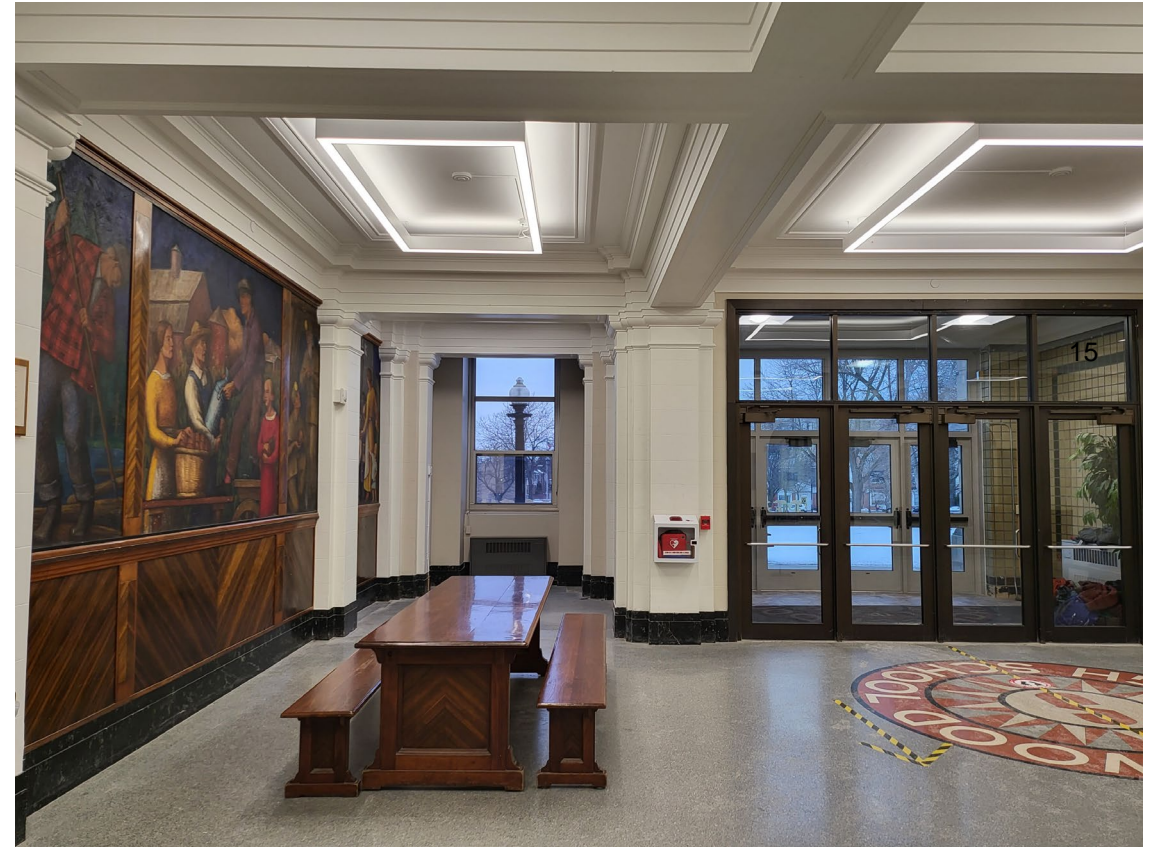
Main entry lobby expanded by removing side offices – increased daylight
