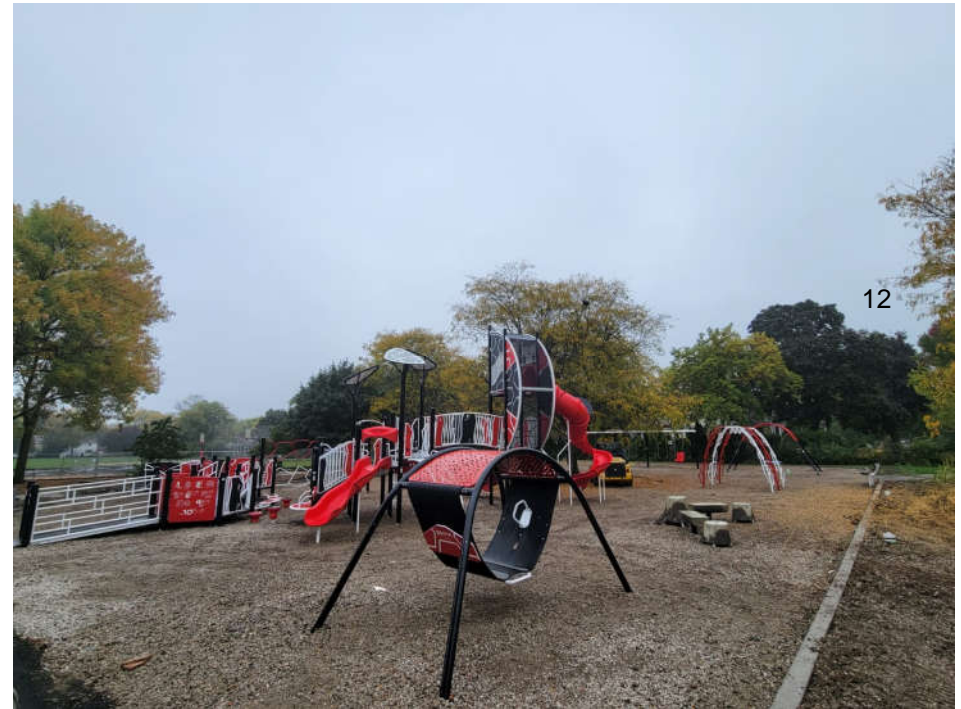
Lake Bluff's North Playground is ready for soft rubber ground surface
