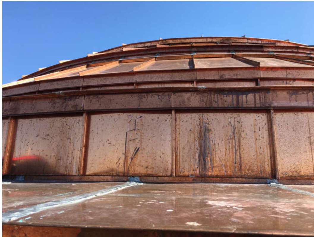
Renovations to the copper dome-exterior
