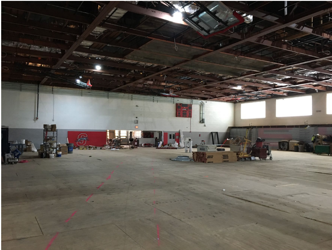
Arena gym is well underway
