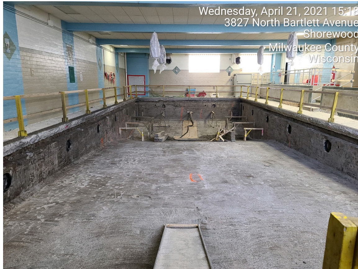
Demolition complete at pool
