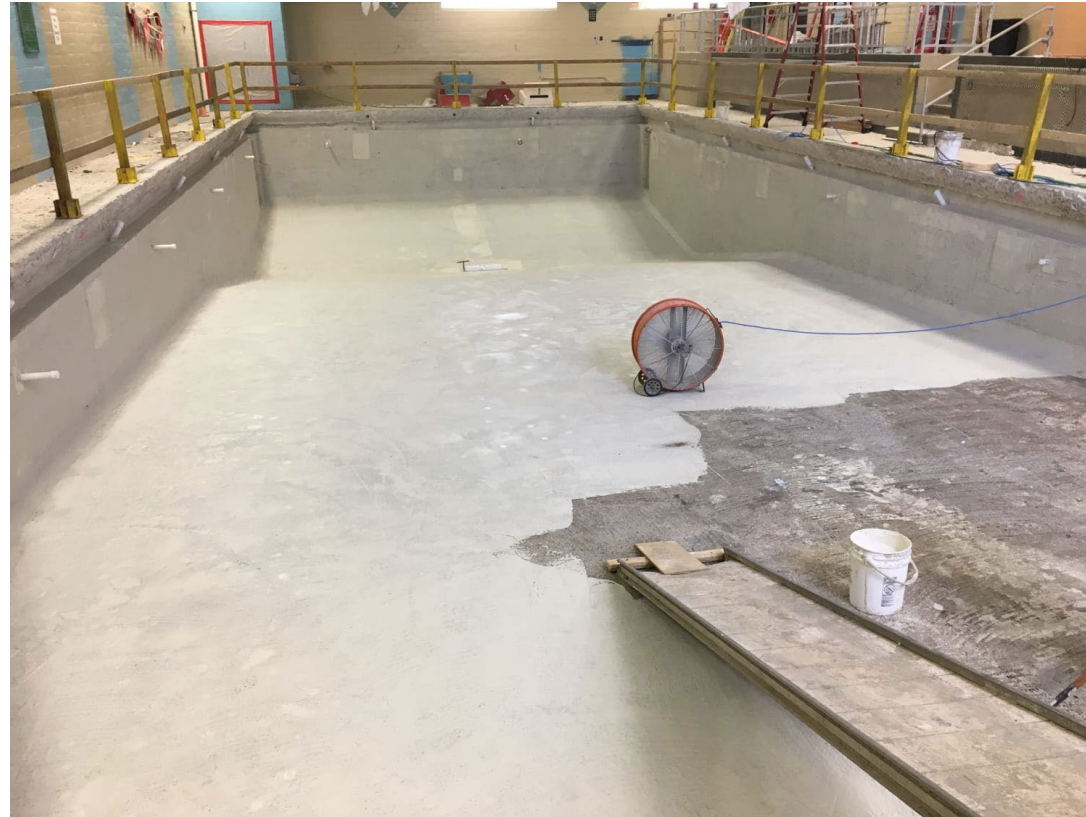
Installation of epoxy coating prior to plaster finish
