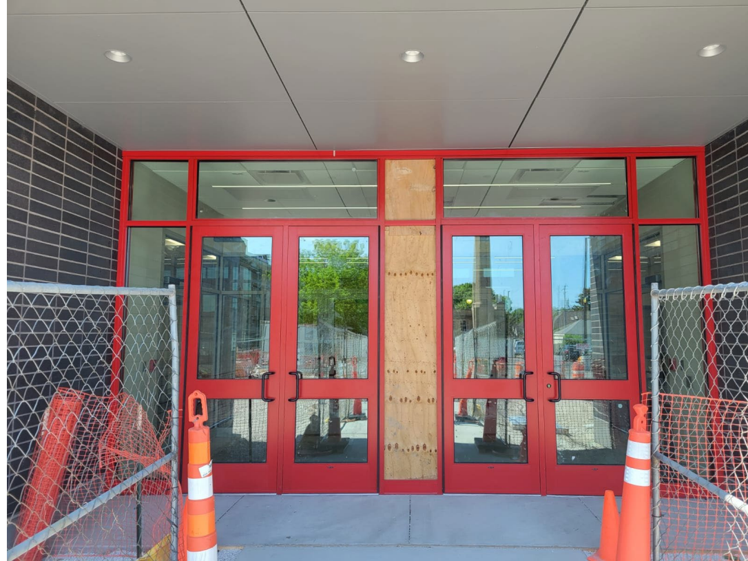
Door frames have been installed at the new admin addition
