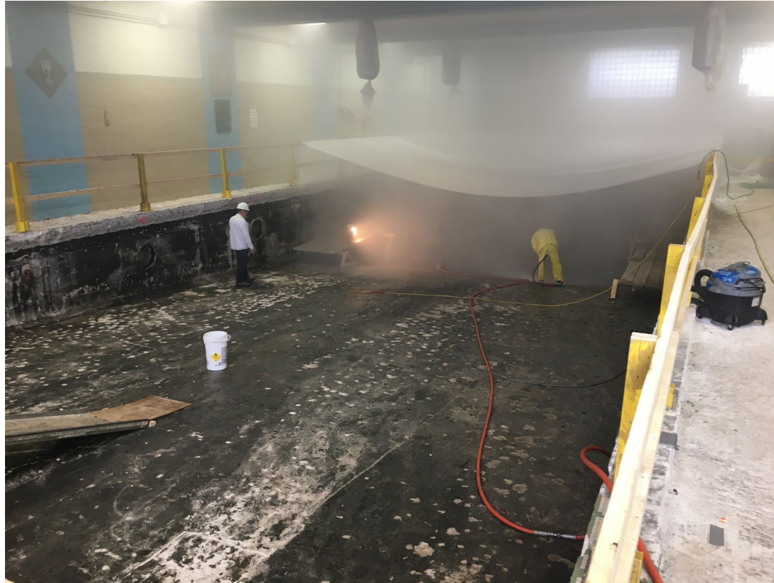
Aggressive power-wash to remove tile mastic
