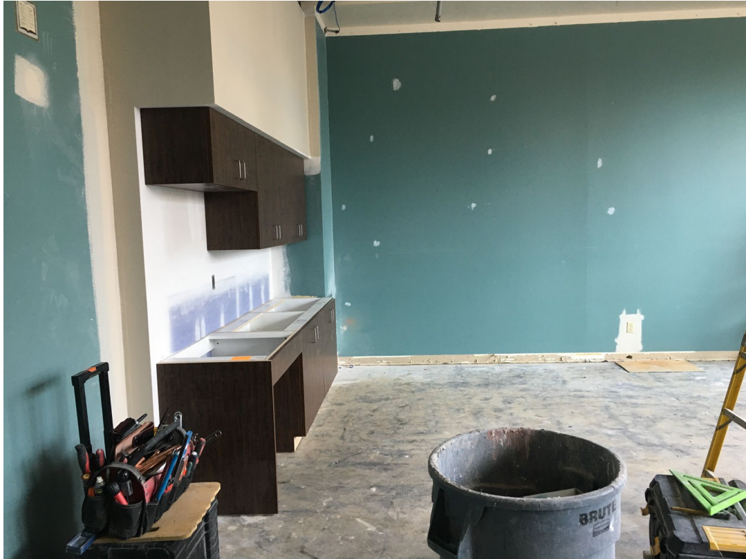
Latest phase of classroom renovation
