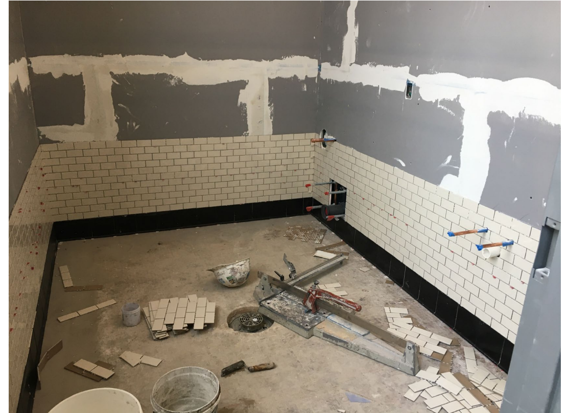
Renovations in restroom
