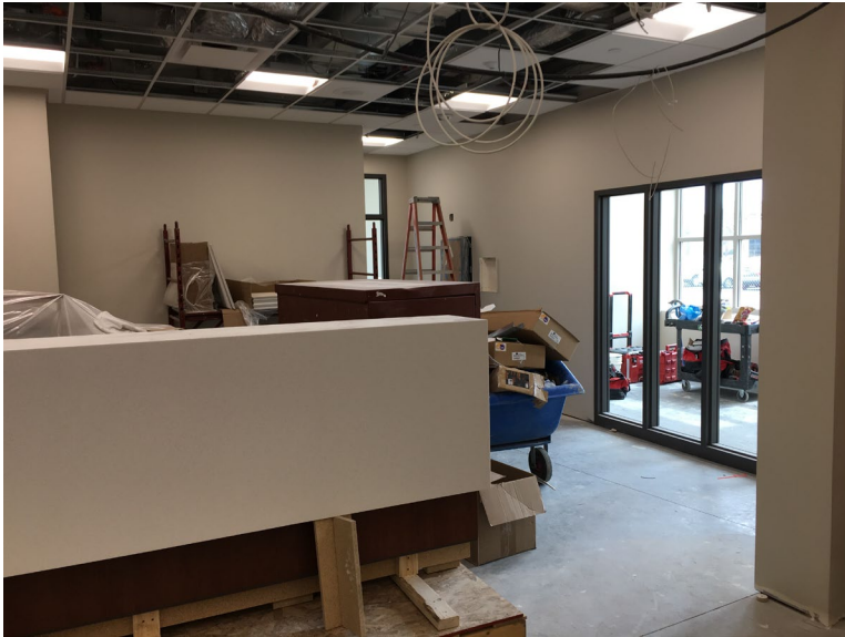
1st floor addition
