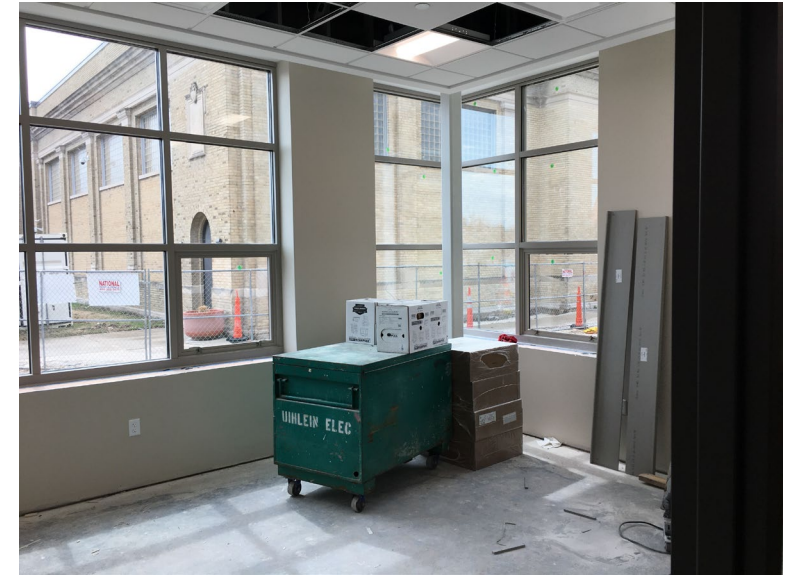
1st floor addition
