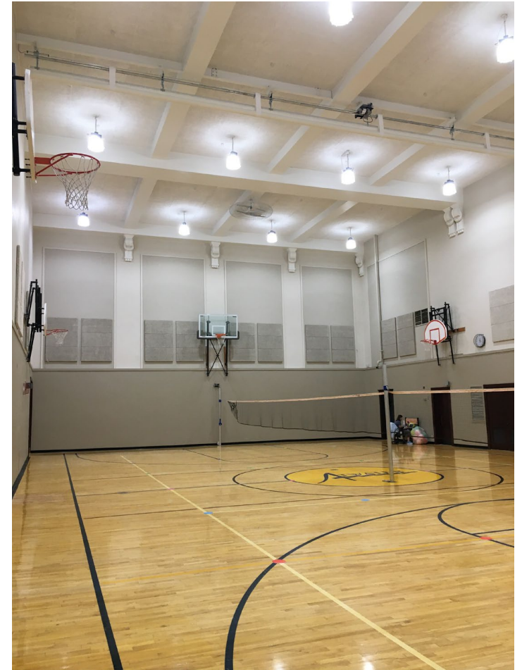
Divider curtain installed - last element of renovated gym
