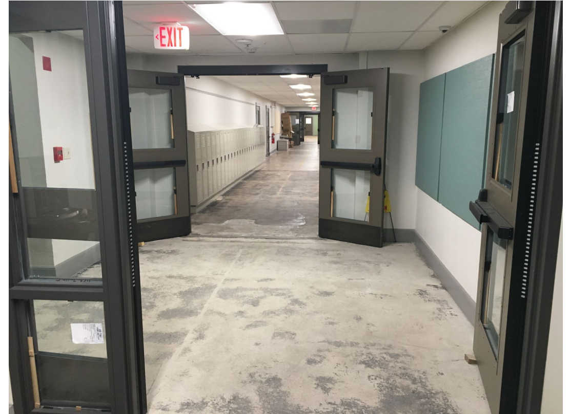
New corridor fire doors and lockers in lower level
