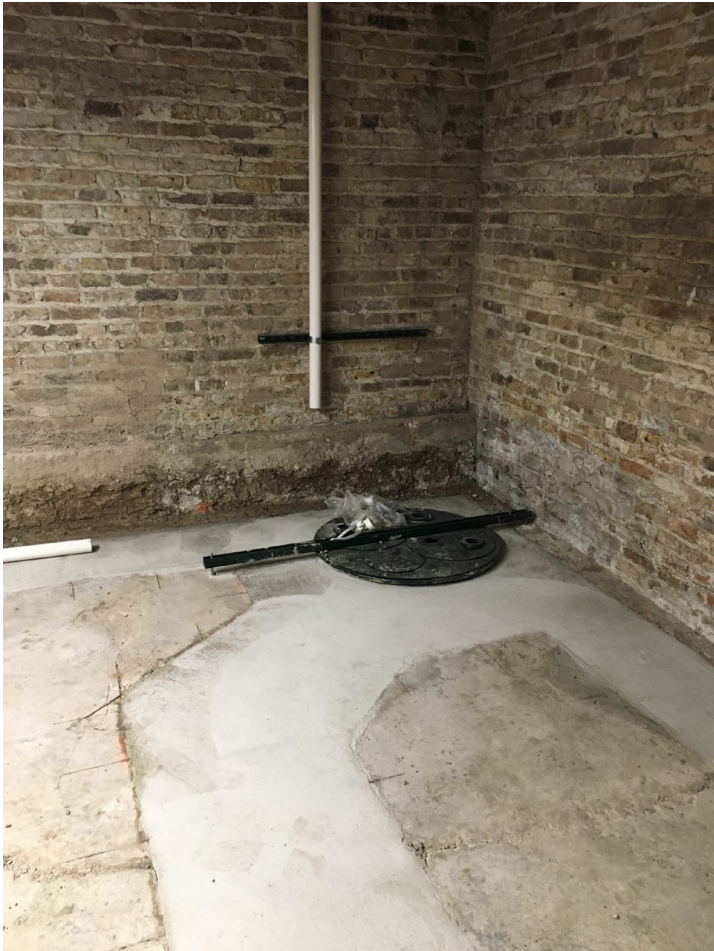
Drain-tile cut into mechanical room floors
