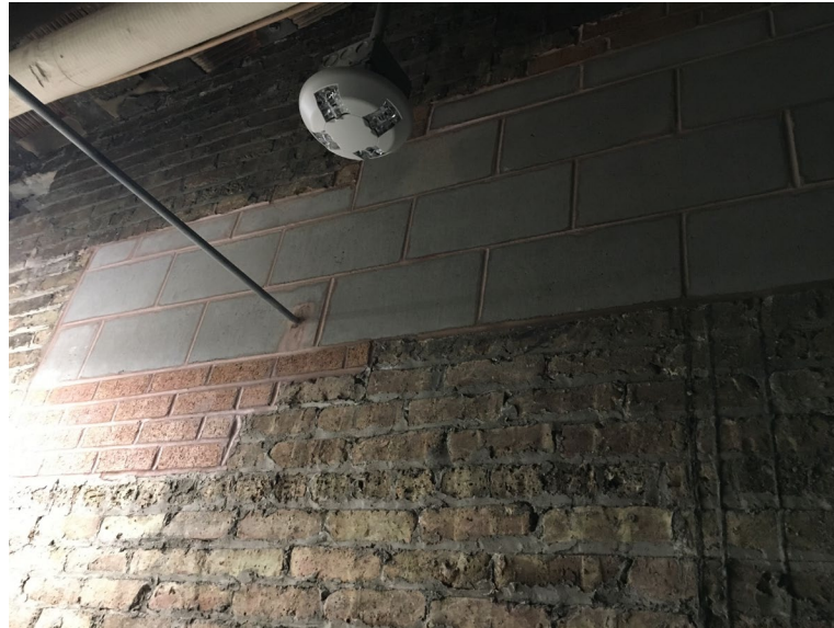
Load bearing walls repaired
