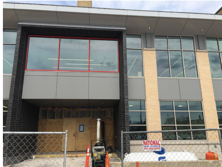
New addition from outside
