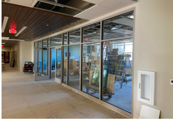
Second Floor "Quiet" Library Entrance
