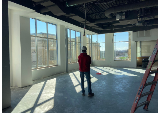
Second Floor addition (facing west)
