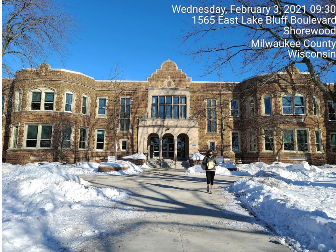
New Window installation is complete
