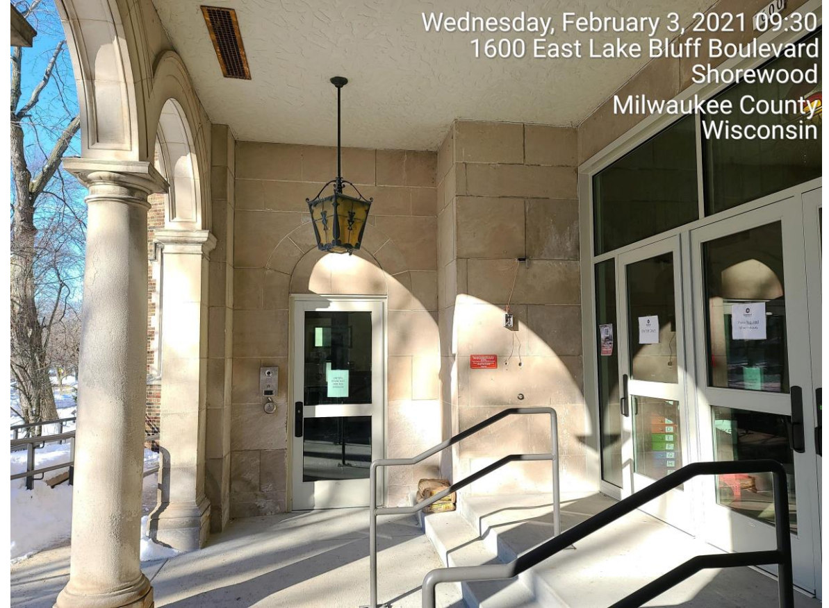
New secure and ADA entrance (exterior)
