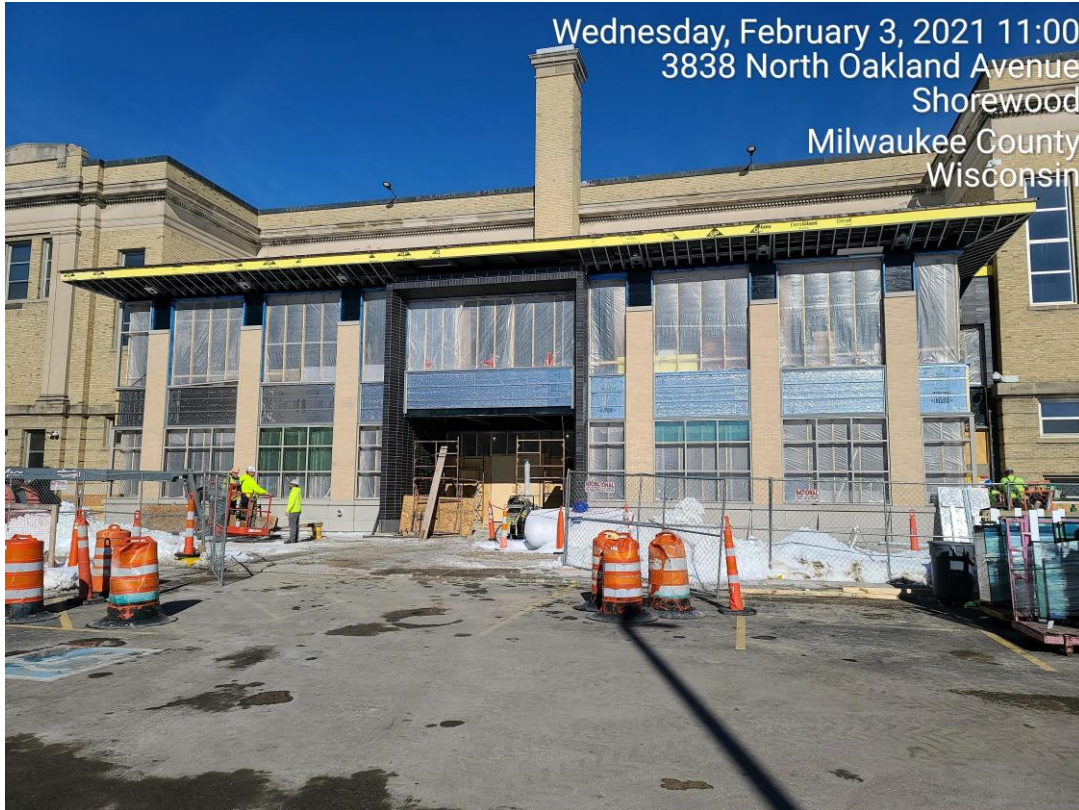
Windows are being installed at the new admin addition
