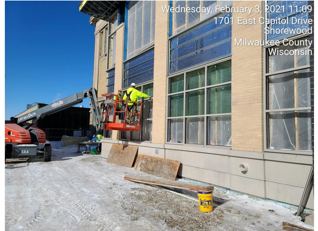
Windows are being installed at the new admin addition
