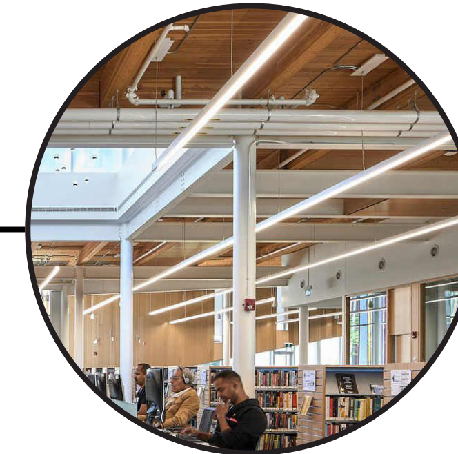
High-Efficiency Light Fixtures and Daylight from Above Reduce Power Demand
