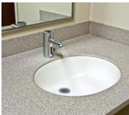
Dual flush toilets and infrared faucets installed at Elgin Academy in Elgin.
