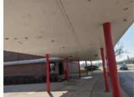
EXISTING CANOPY UNDER SIDE - 3
