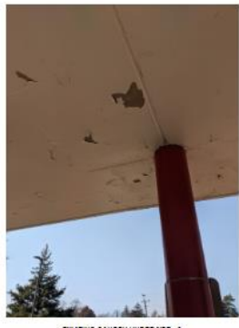
EXISTING CANOPY UNDER SIDE - 2
