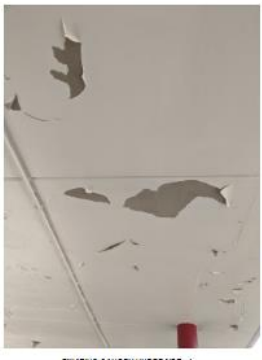
EXISTING CANOPY UNDER SIDE - 1
