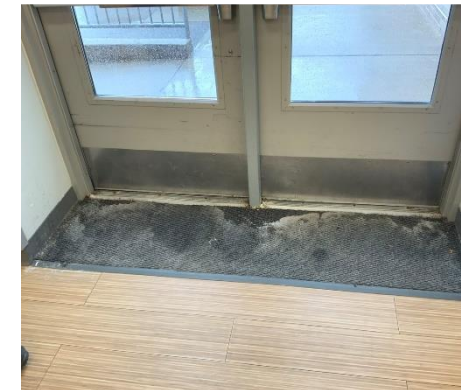
Receiving doors- Adequacy
