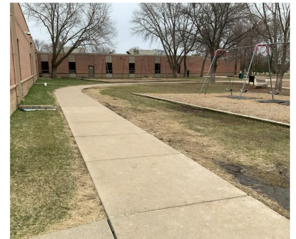
Drainage- Southeast side
