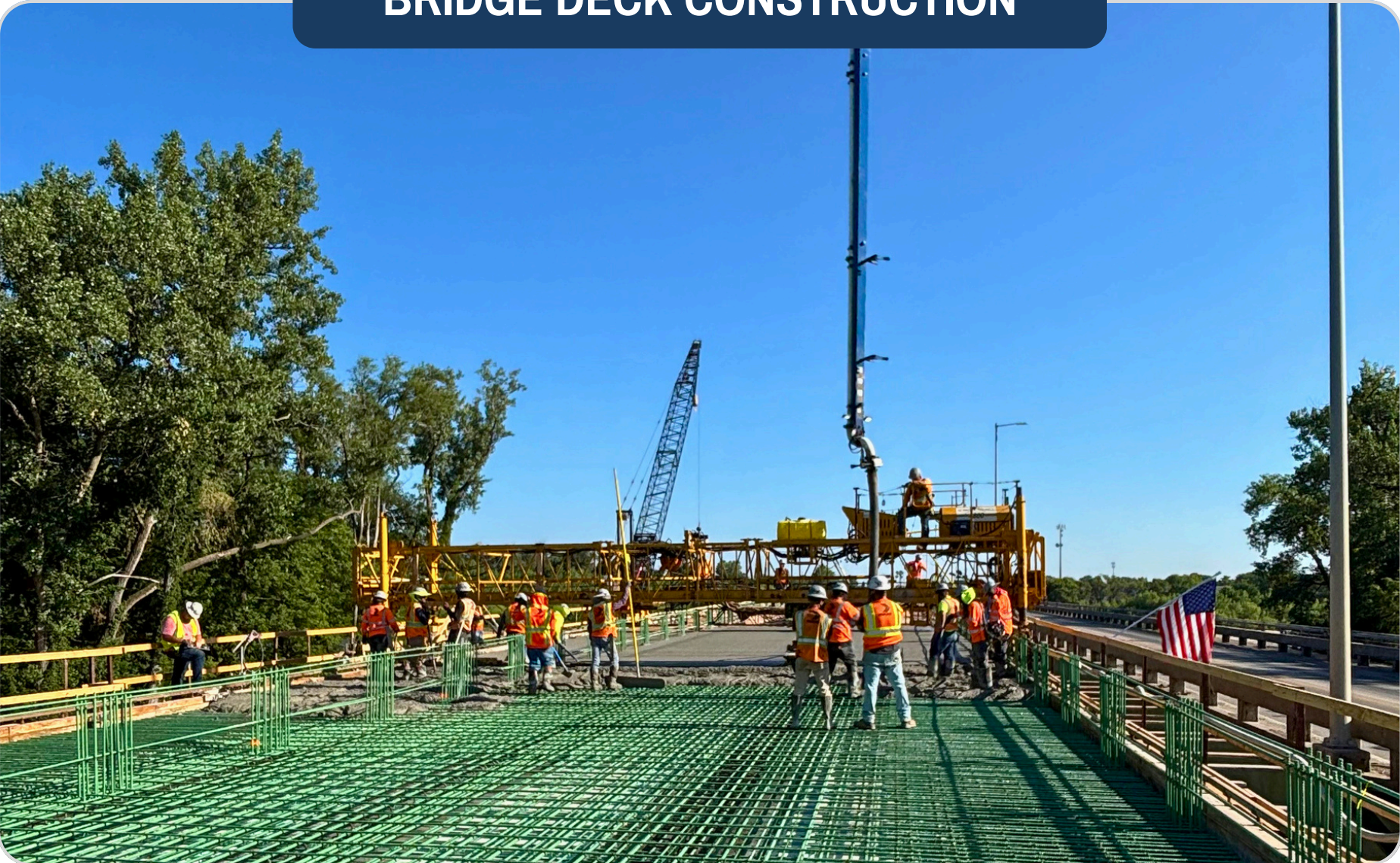
BRIDGE DECK CONSTRUCTION
