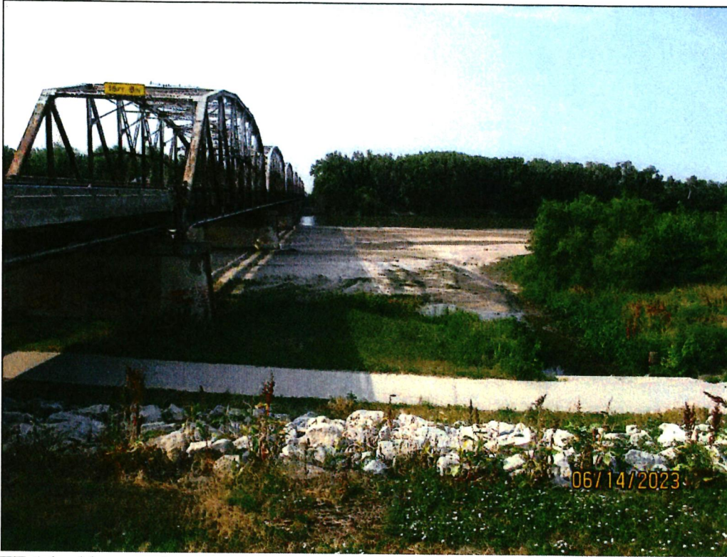
TE 1 looking south
