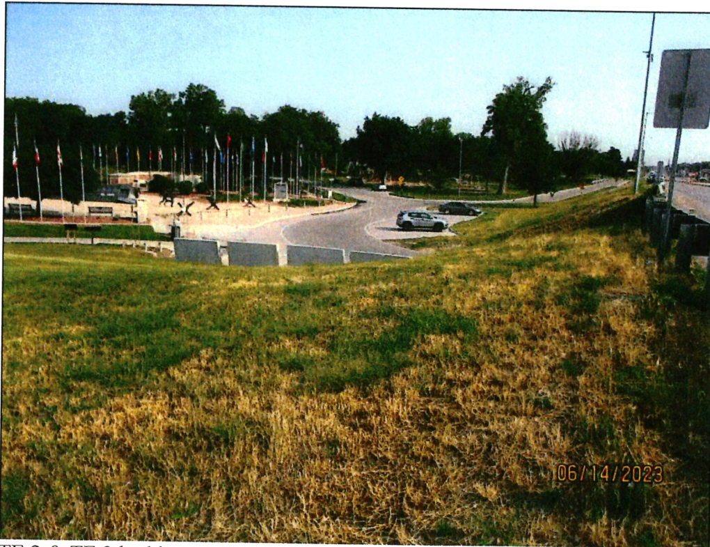
TE 2 & TE 3 looking north
