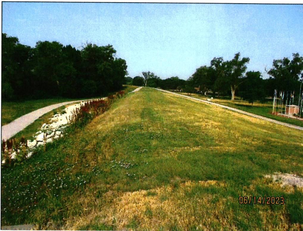
TE 2 looking west
