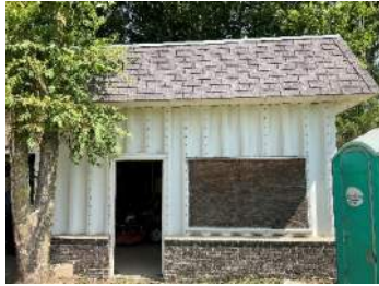
Existing Building Exterior
