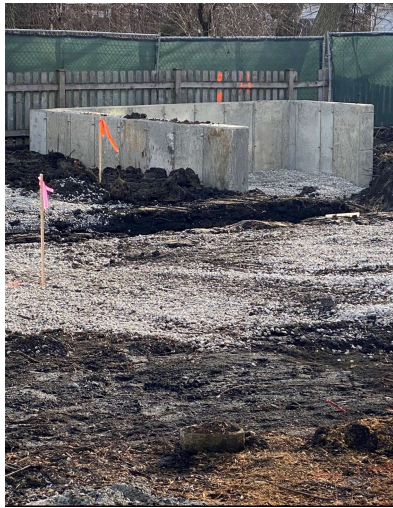
Construction of Retaining Wall
