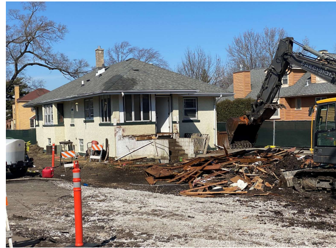
Demolition of Deck/ Garage - Loudon House
