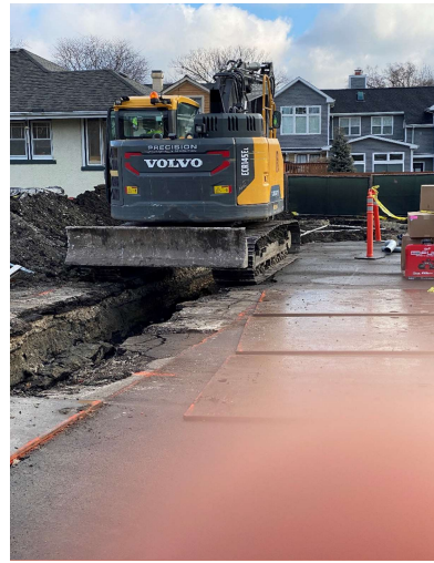
Excavation for ComEd Utilities
