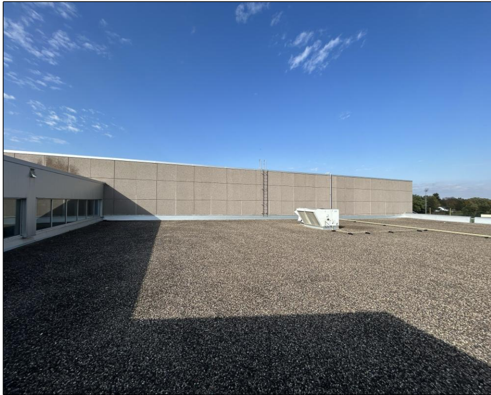
Control joint replacement overview photo.
