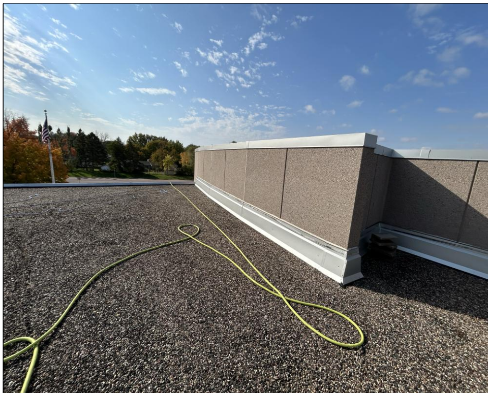
Additional repair location overview.
