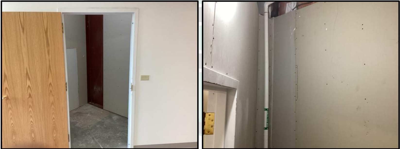
After: Sheetrocked wall and added light fixture and switch in each.
