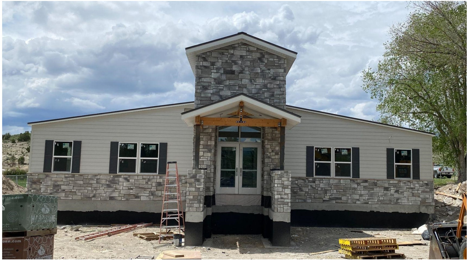
Front Entrance, Roadside view
