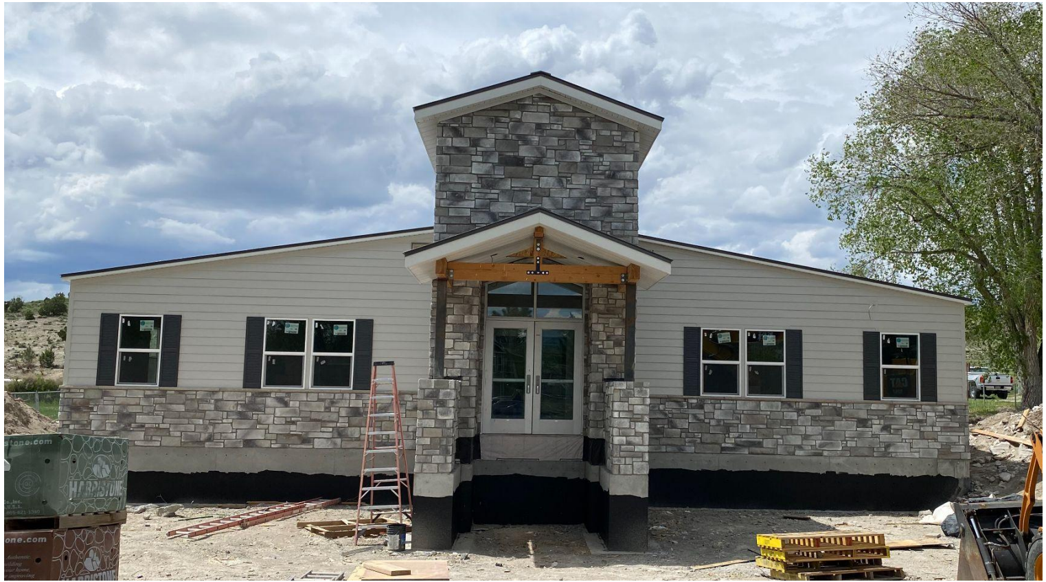
Front Entrance, Roadside view
