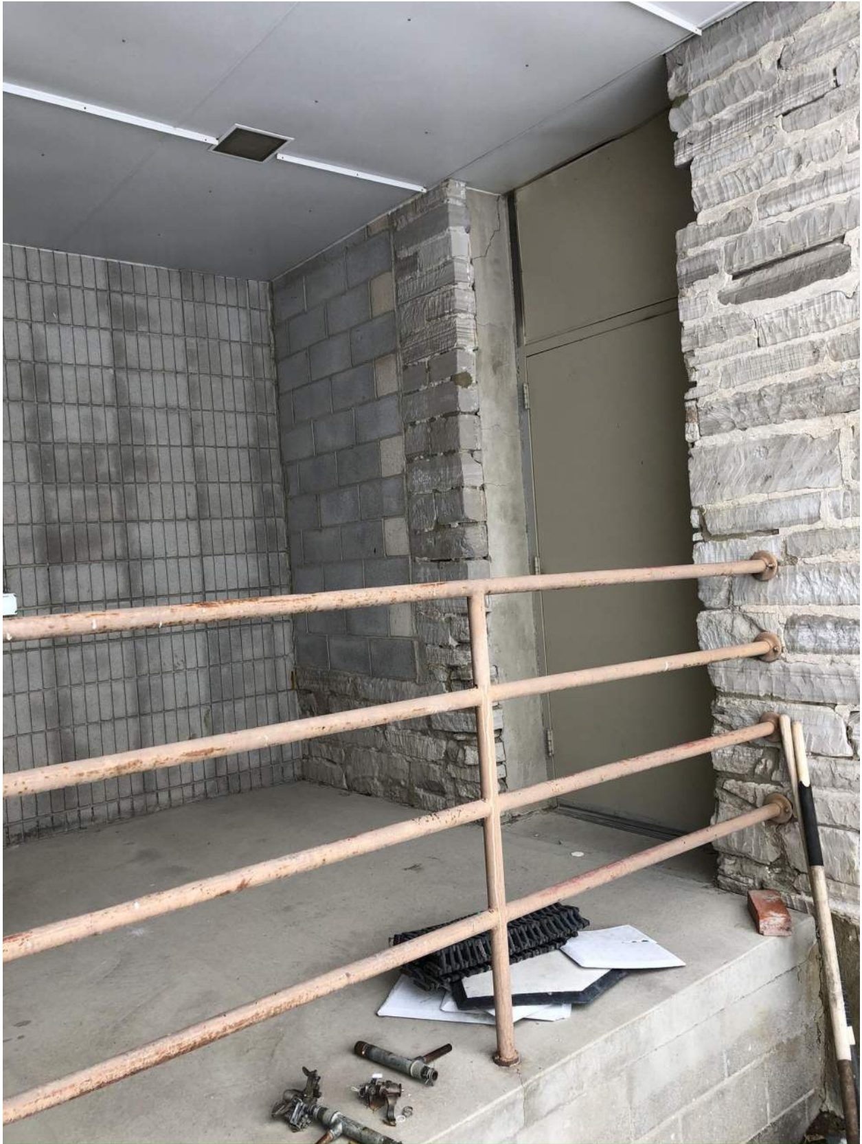
Photo 17 – View of infilled opening in west exterior wall at the Breezeway.
