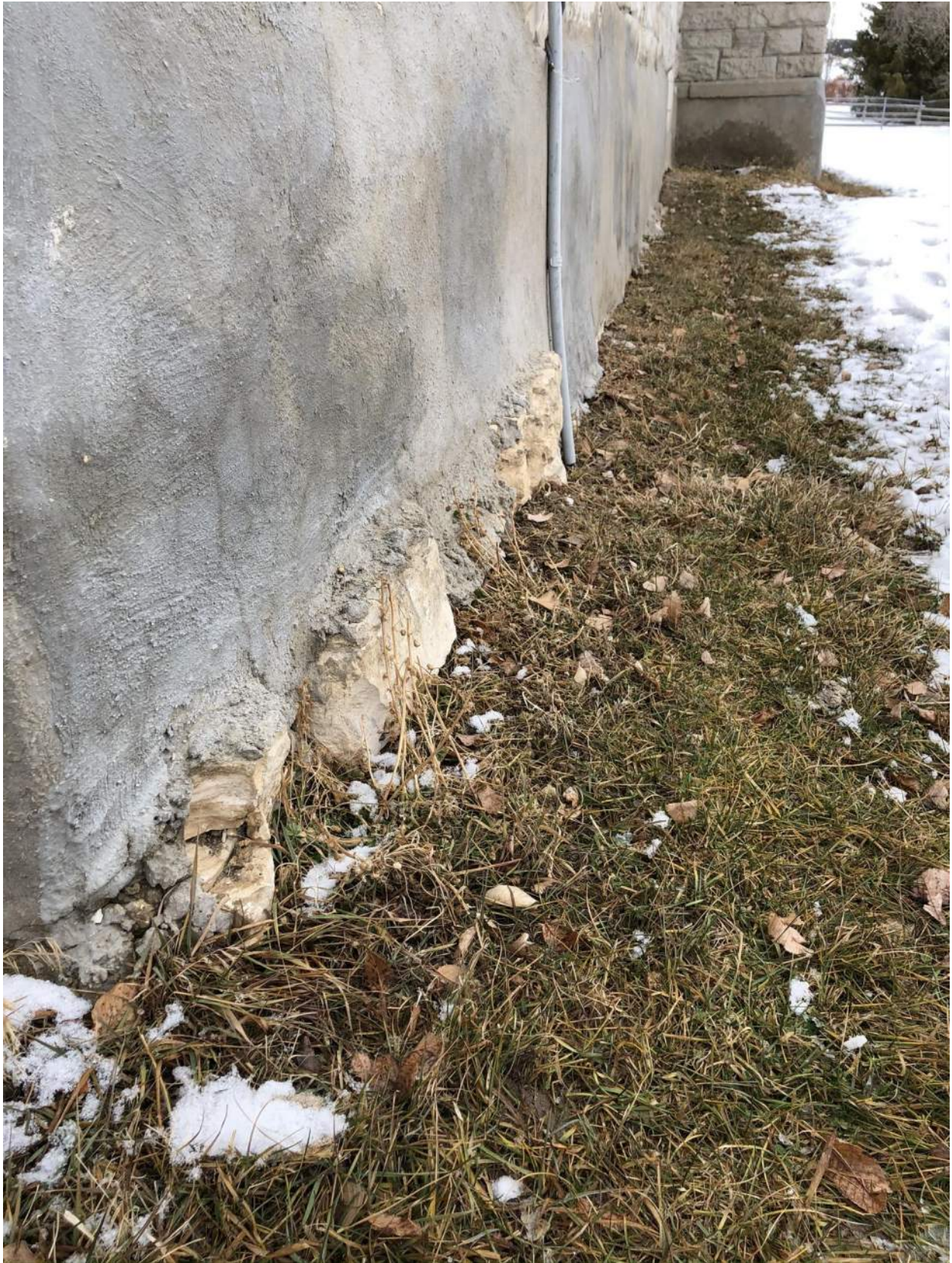
Photo 14 – Another view of the foundation along the south wall. Plastered stone.
