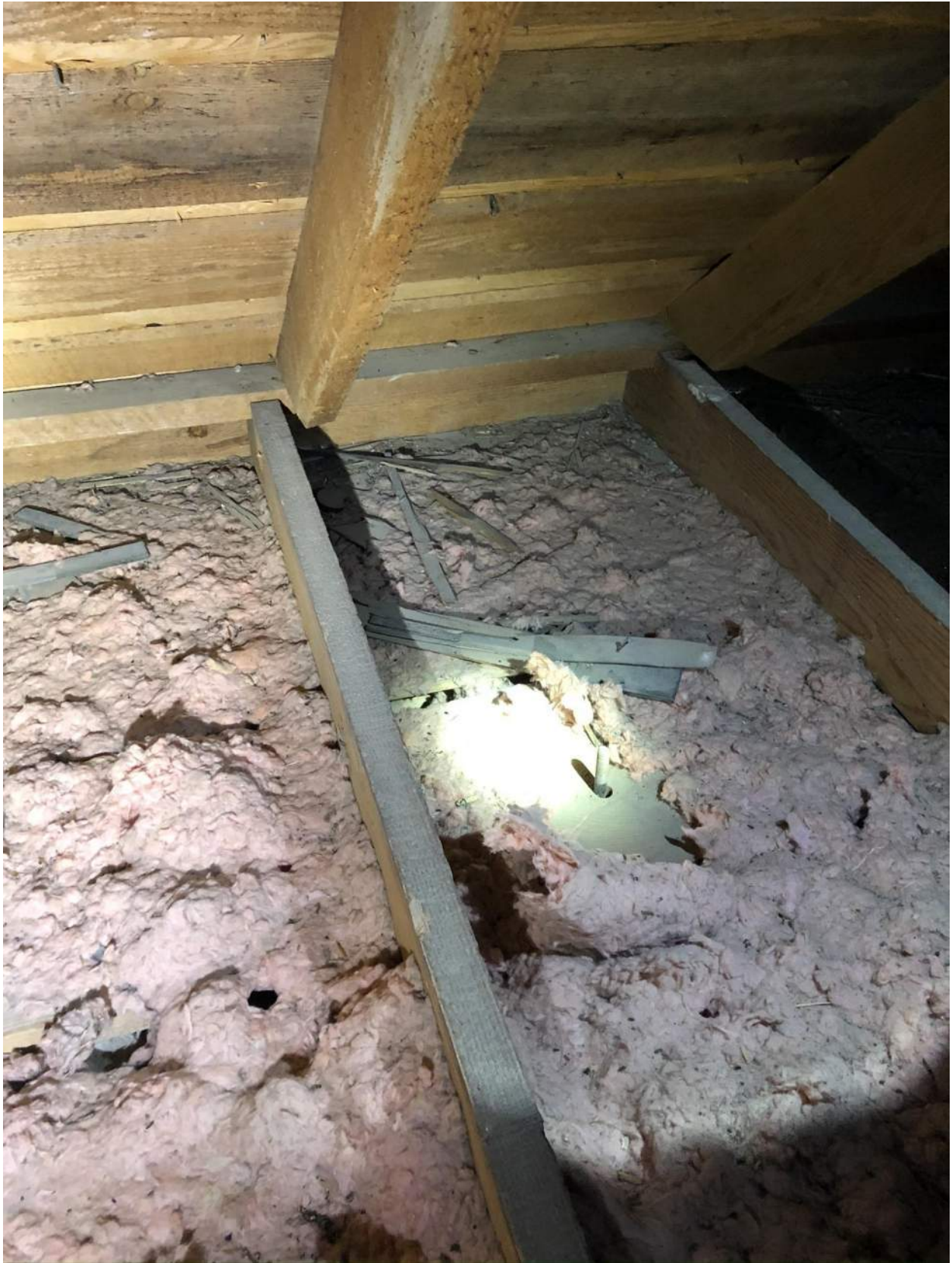
Photo 11 – View of existing anchor bolts along top of stone exterior walls. Bolt locations are erratic. Not nuts or washers are present on the anchor bolts.
