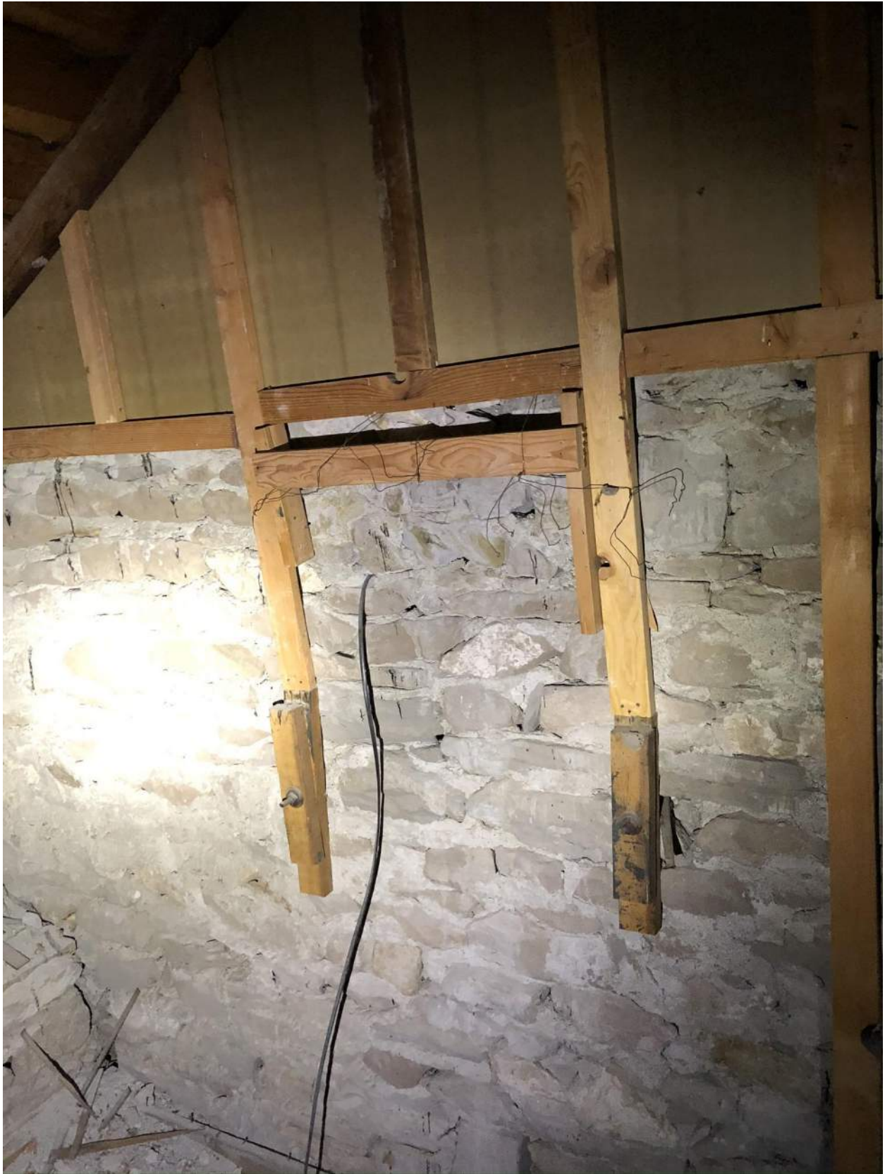
Photo 9 - View of inside face of gabled end wall above east entry. This shows how the wood canopy is anchored.
