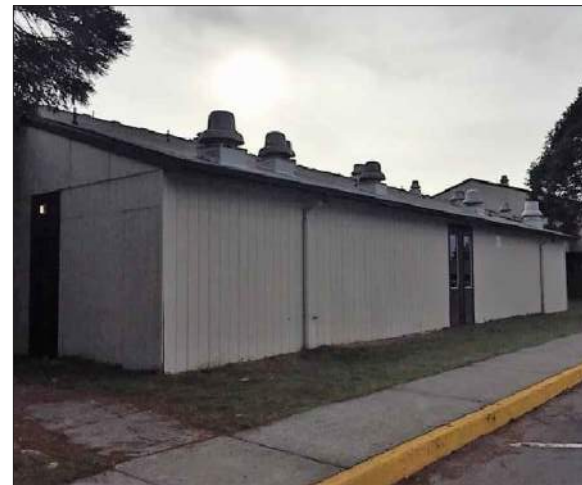
VIEW F LOOKING SOUTHEAST AT CLASSROOM WING
