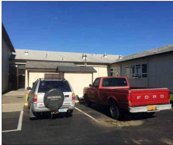
VIEW A LOOKING NORTH AT BUILDING D CONNECTION TO ORIGINAL HIGH SCHOOL BUILDING
