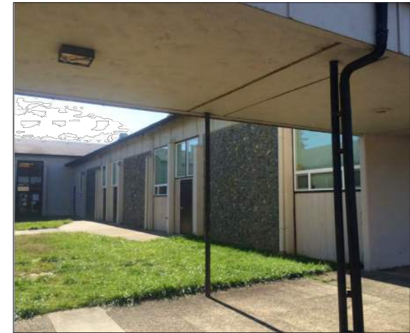
VIEW D LOOKING SOUTHWEST AT CLASSROOM WING
