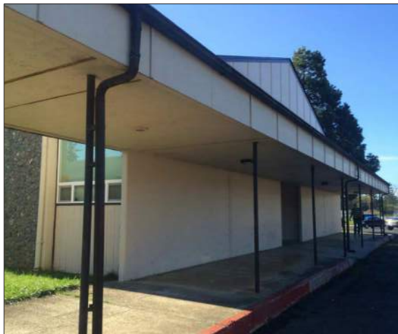
VIEW E LOOKING SOUTHWEST AT CLASSROOM WING
