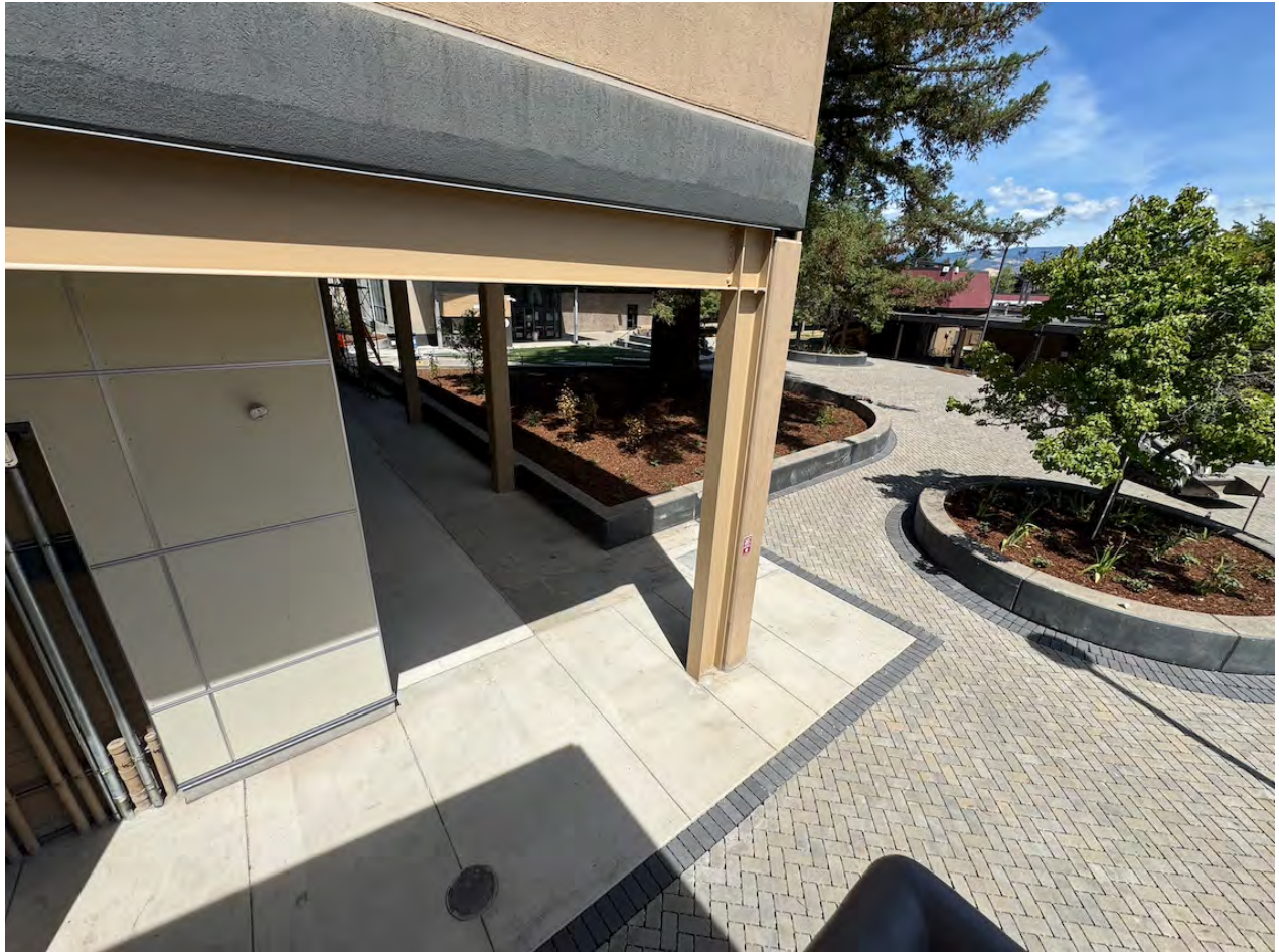
Interface of Seismic Structural Members, Quad Renovation and New Cladding
