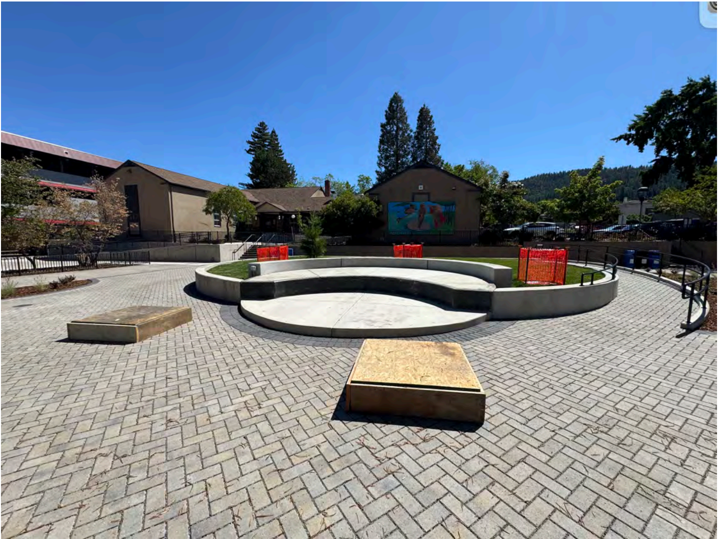
South Facing View of the Quad Renovations
