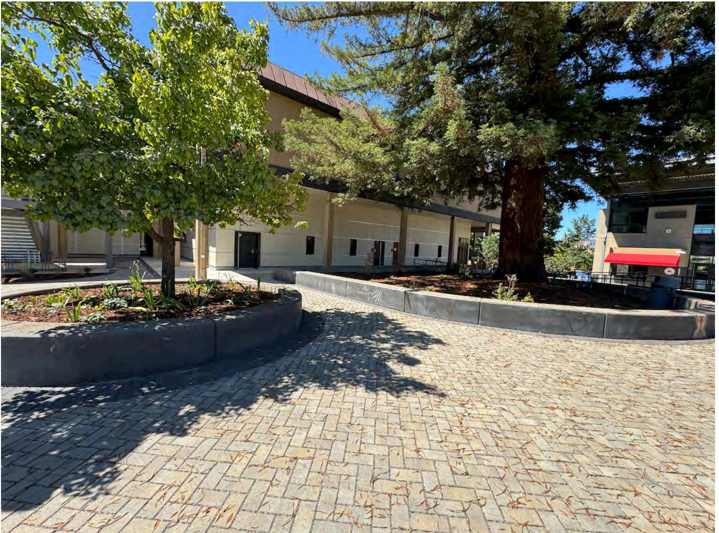
Renovated Science Building with a partial glimpse at the quad upgrades in the foreground
