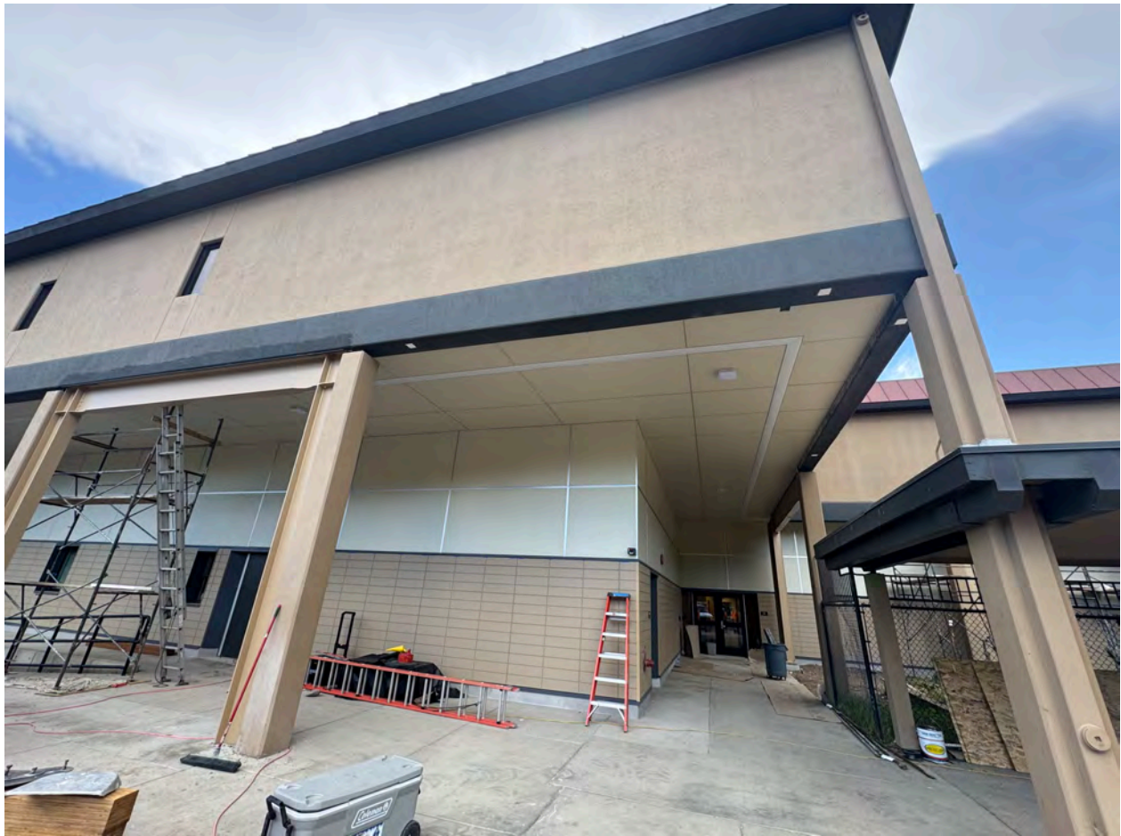
AHS Science Building Revealing New Concrete, Siding, Soffit and Structural Upgrades!
