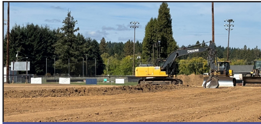
Fields Project - Grading Underway
