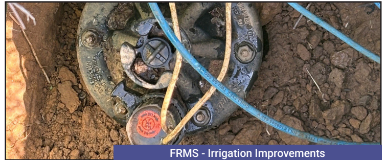
FRMS - Irrigation Improvements
