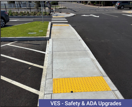
VES - Safety & ADA Upgrades
