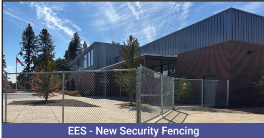
EES - New Security Fencing
