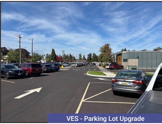
VES - Parking Lot Upgrade
