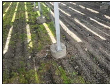
Concrete pier & anchors.
