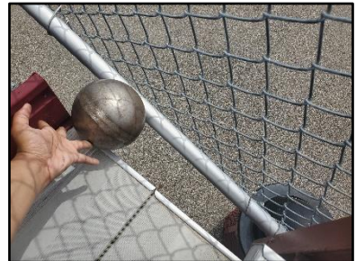
Proper guardrail gap closure.
