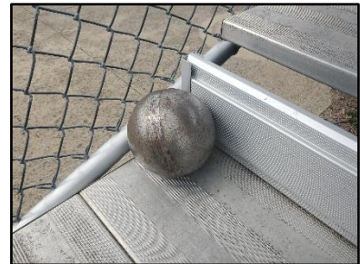
Proper guardrail gap closure.
