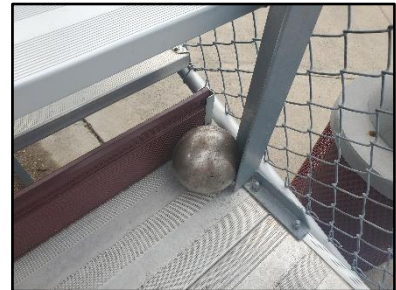
Proper guardrail gap closure.
