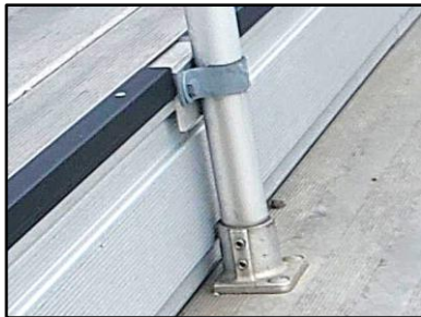
Handrail anchor attachment.
