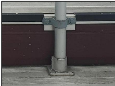
Handrail anchor attachment.
