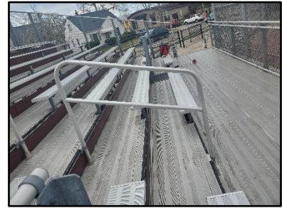
Mid aisle handrail.
