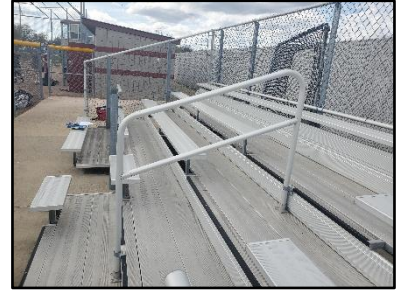
Mid aisle handrail.
