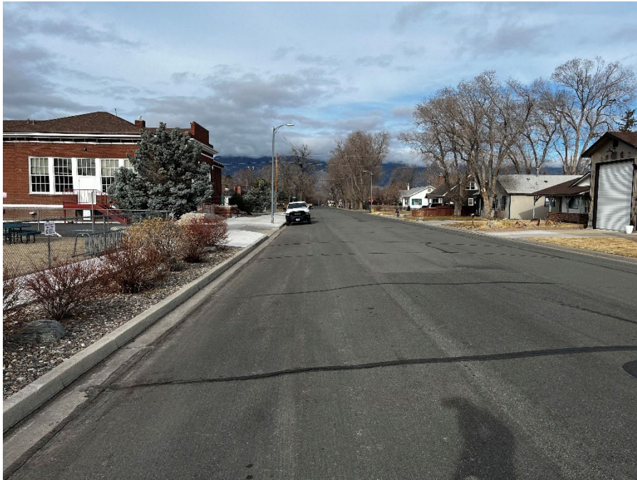
VIEW LOOKING WESTERLY ALONG MONO AVENUE ADJACENT TO SUBJECT PROPERTY
