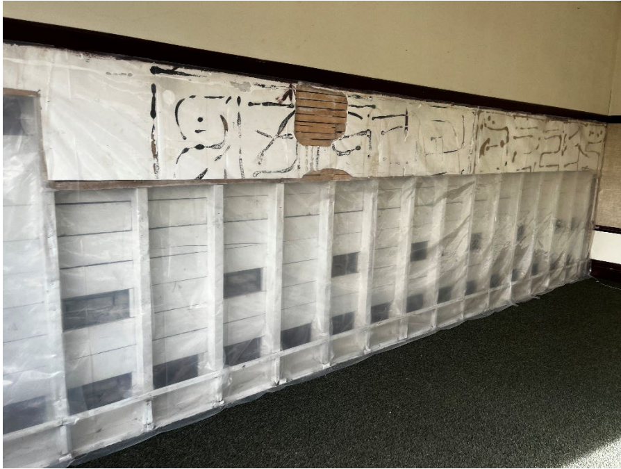
VIEW OF REMEDIATION WORK ON EXTERIOR FACING WALL
