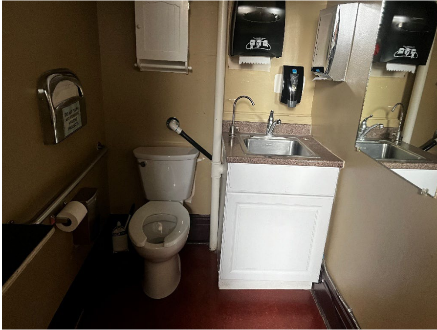
VIEW OF SINGLE RESTROOM ON MAIN LEVEL
