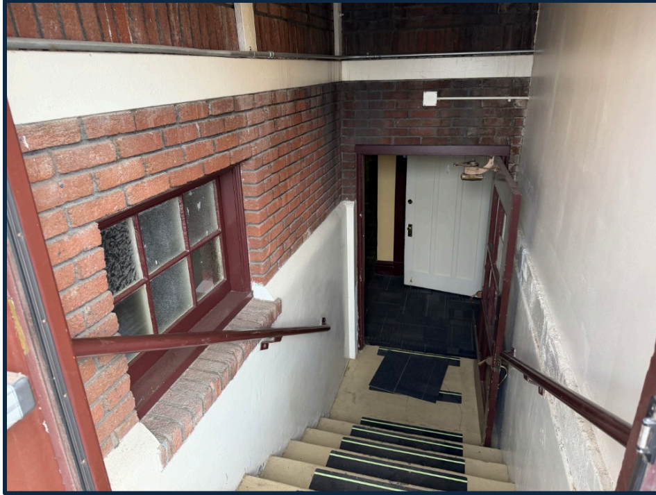
Subject basement access
