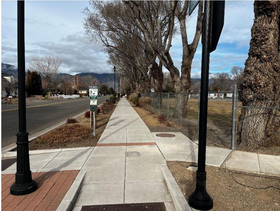
VIEW LOOKING WESTERLY ALONG THE WALKING PATH ON THE SUBJECT'S FRONTAGE ON COUNTY ROAD
