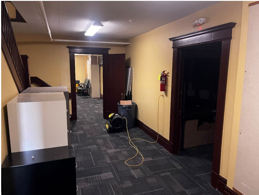
VIEW OF CORRIDOR ON BASEMENT LEVEL
