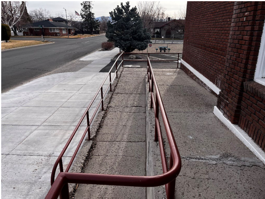
VIEW OF RAMP TO MAIN ENTRANCE
