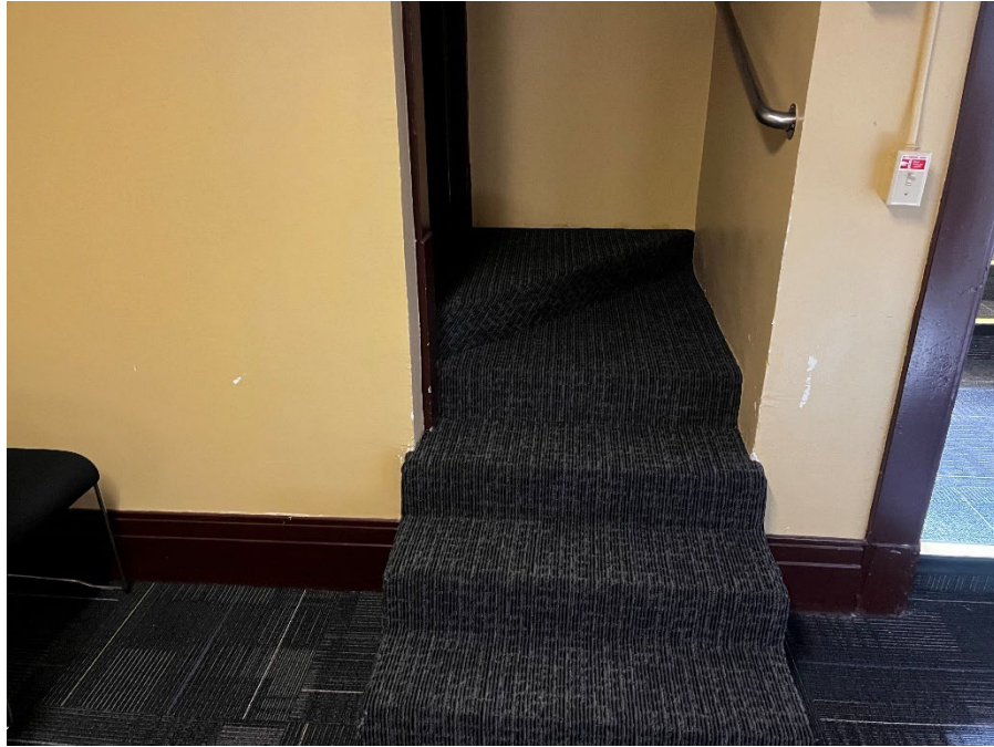
VIEW OF ENTRANCE TO RESTROOM ON BASEMENT LEVEL
