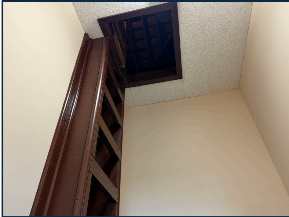
Subject roof access
