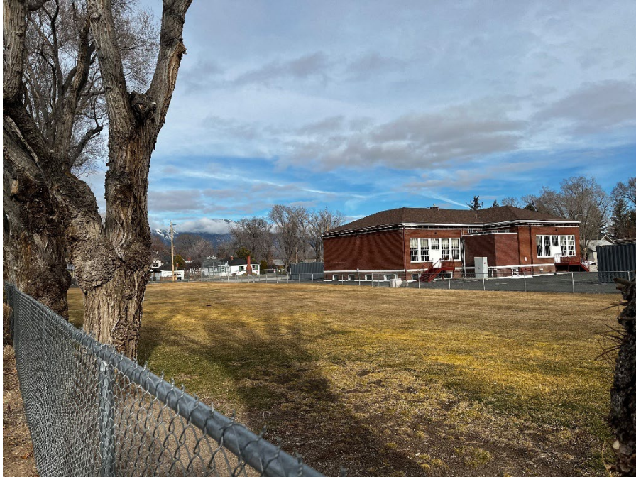
VIEW LOOKING NORTHWESTERLY ACROSS THE PARCEL
