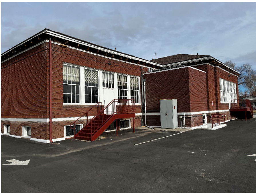
VIEW LOOKING NORTHEASTERLY AT THE SOUTHERN FACE OF THE SUBJECT PROPERTY
