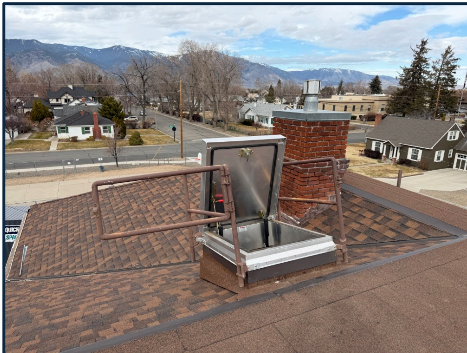
Subject roof hatch
