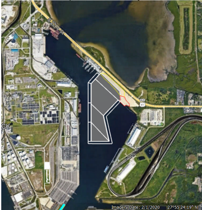
Eastport Future Fill Project
