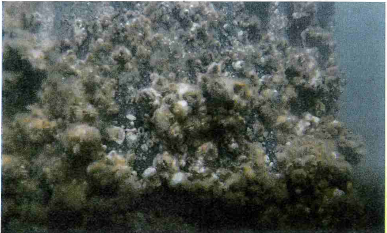
Photo 3: Typical view of barnacle-encrusted dock piling
