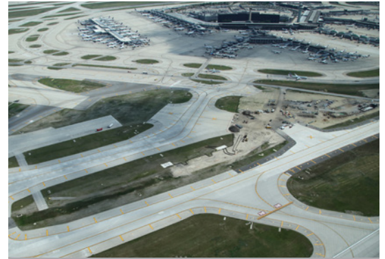
CONSTRUCTION TYPE: New Construction
