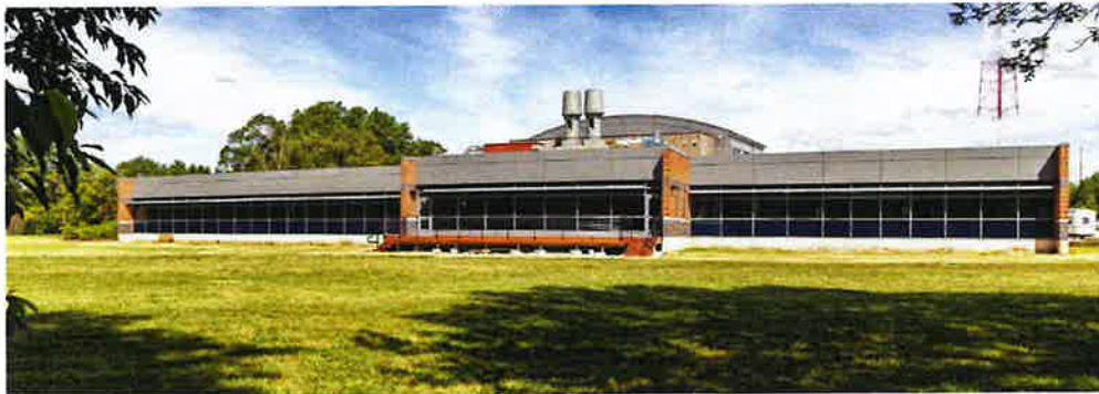
Fox River Water Reclamation District
